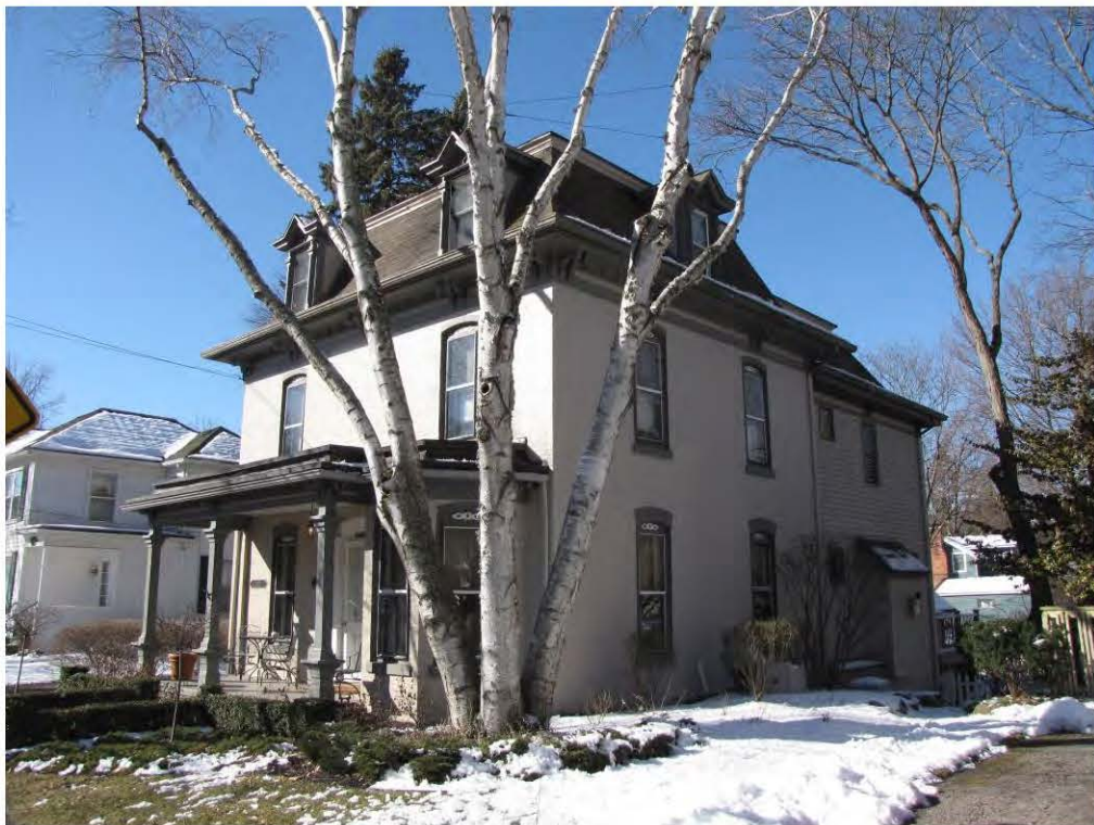
Rogers North 109_Looking Southwest
