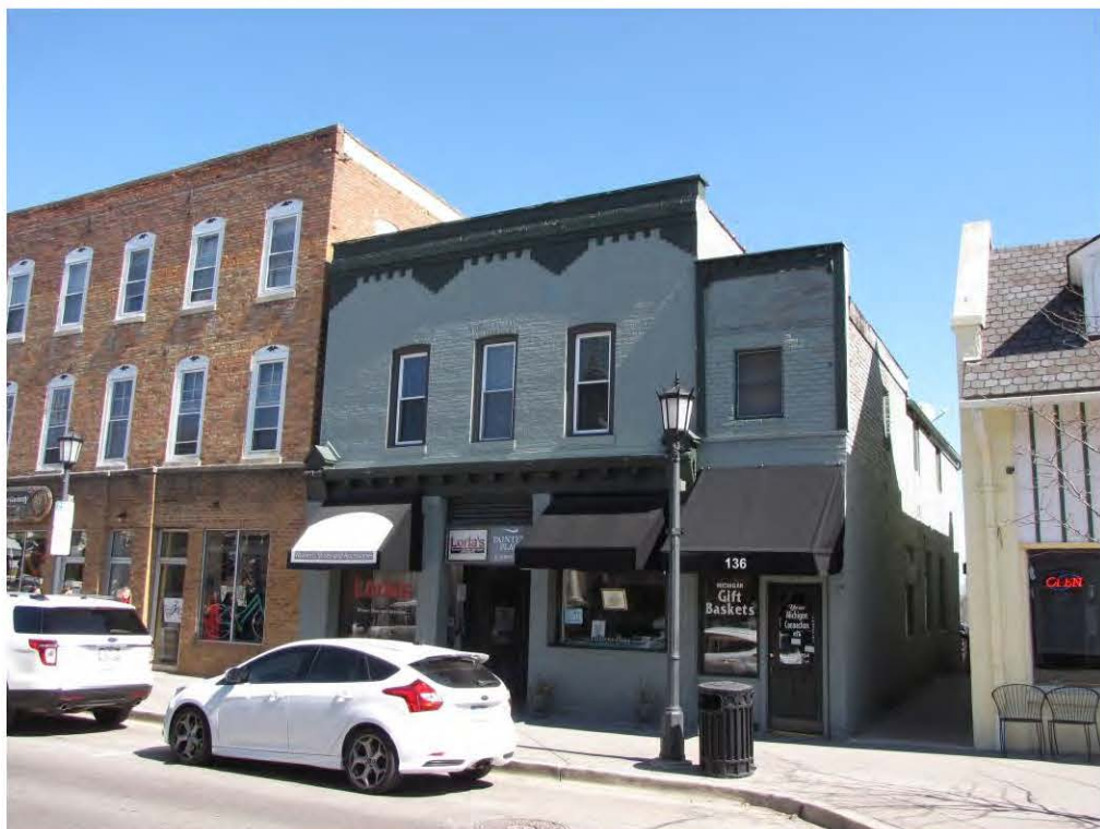
Center North 136-142_Looking Northeast
