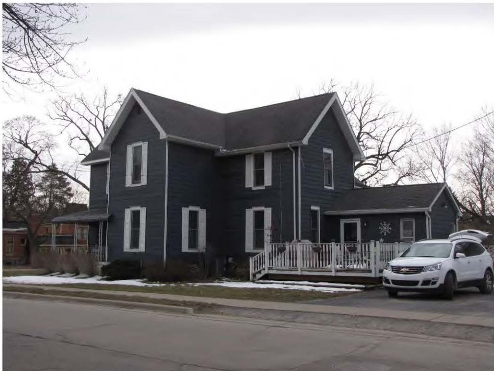
Rogers South 102_Looking Southeast
