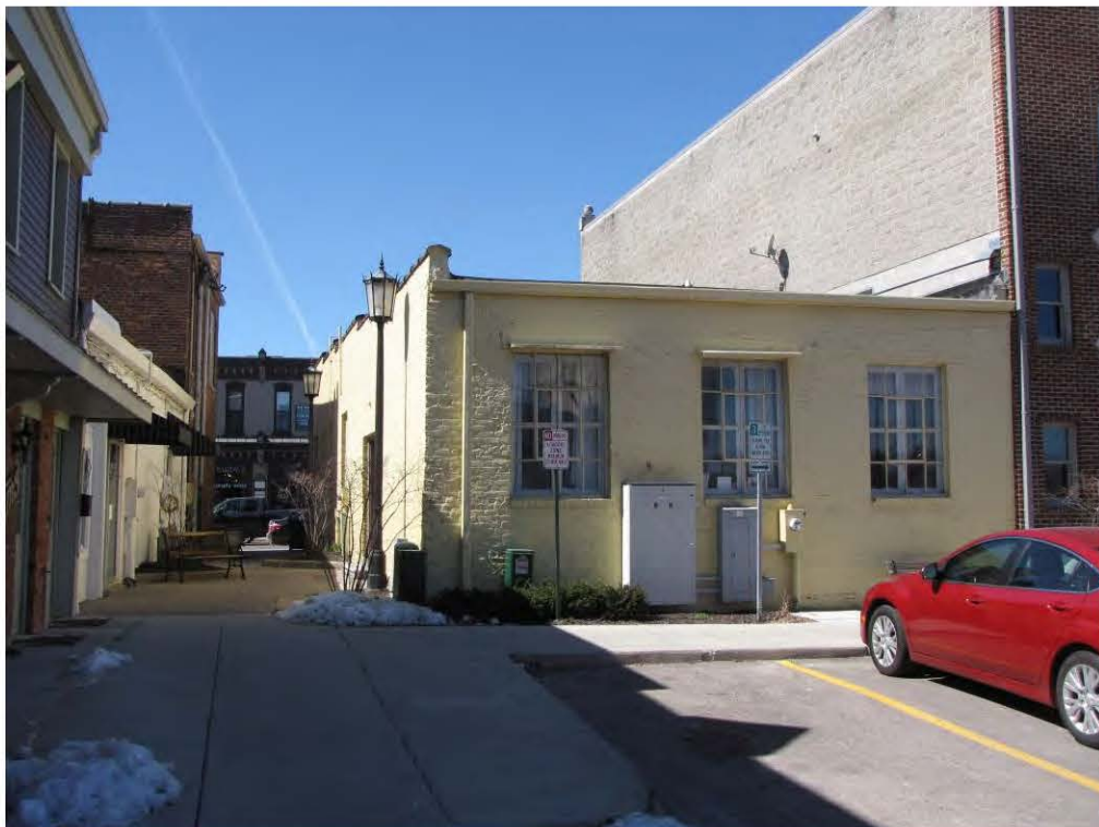
Center North 120_Looking West
