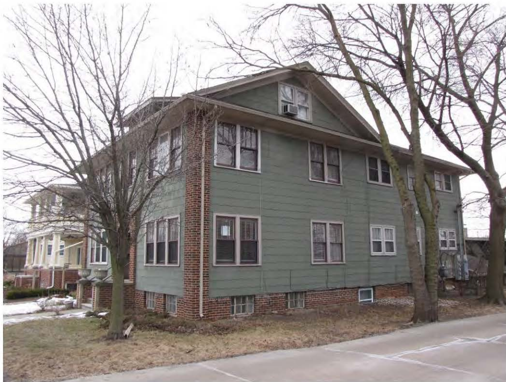
Main East 430_Looking Southeast
