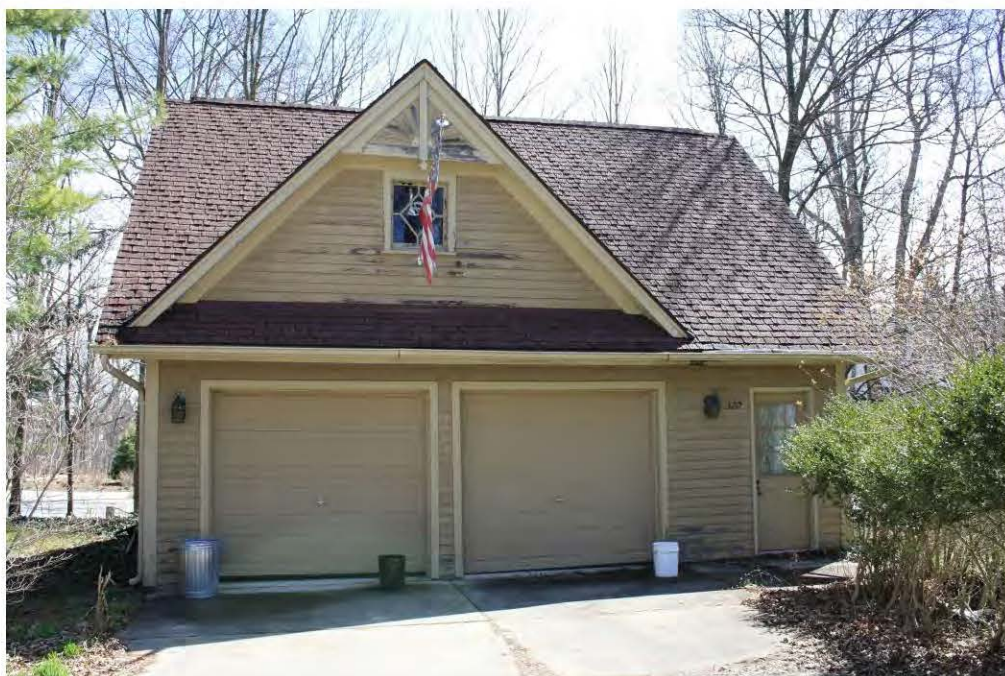
High 320, Garage_Looking East
