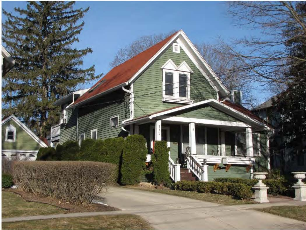
Rogers North 359_Looking Northwest
