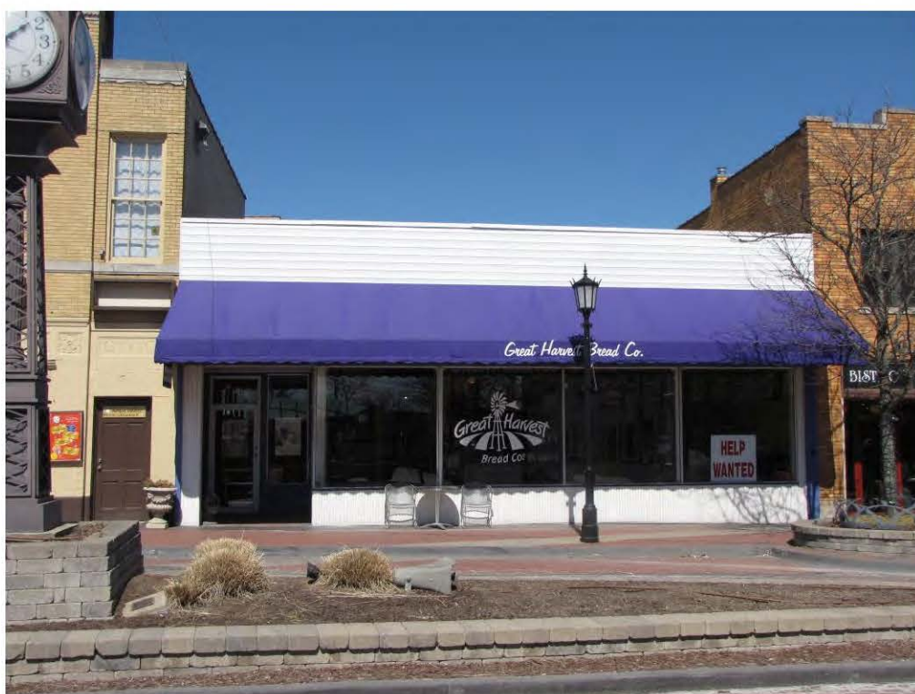
Main East 139_Looking North
