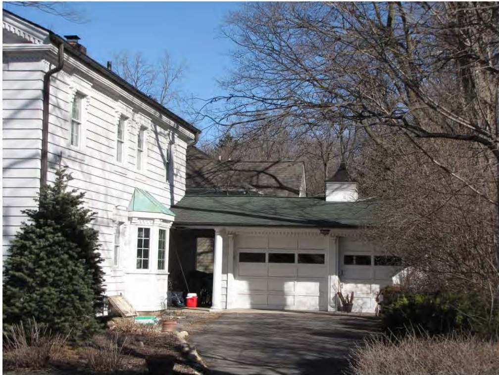
Randolph 204, Garage_Looking North
