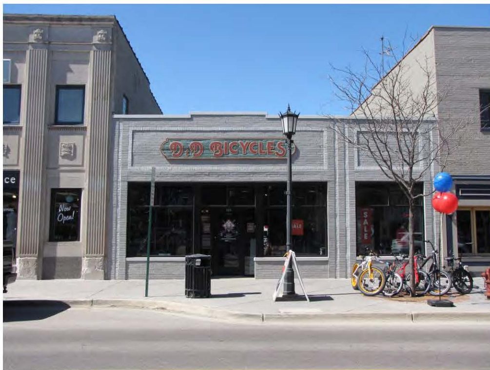
Center North 121_Looking West
