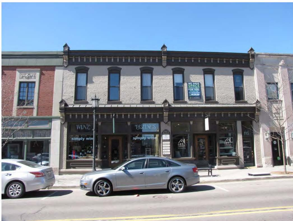
Center North 109-115_Looking West
