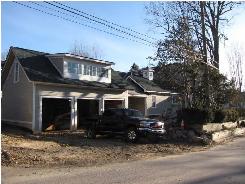
Rogers North 333_Looking Northeast
