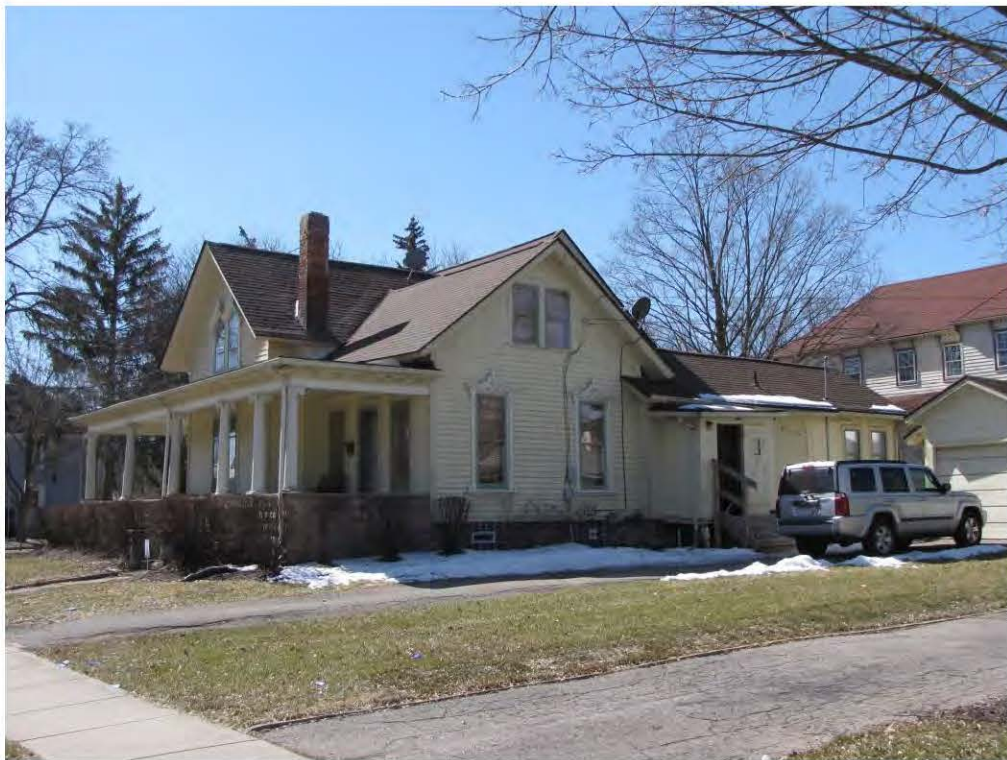
Dunlap West 304_Looking Southwest
