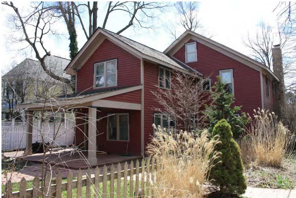
Dunlap West 418_Looking Southeast
