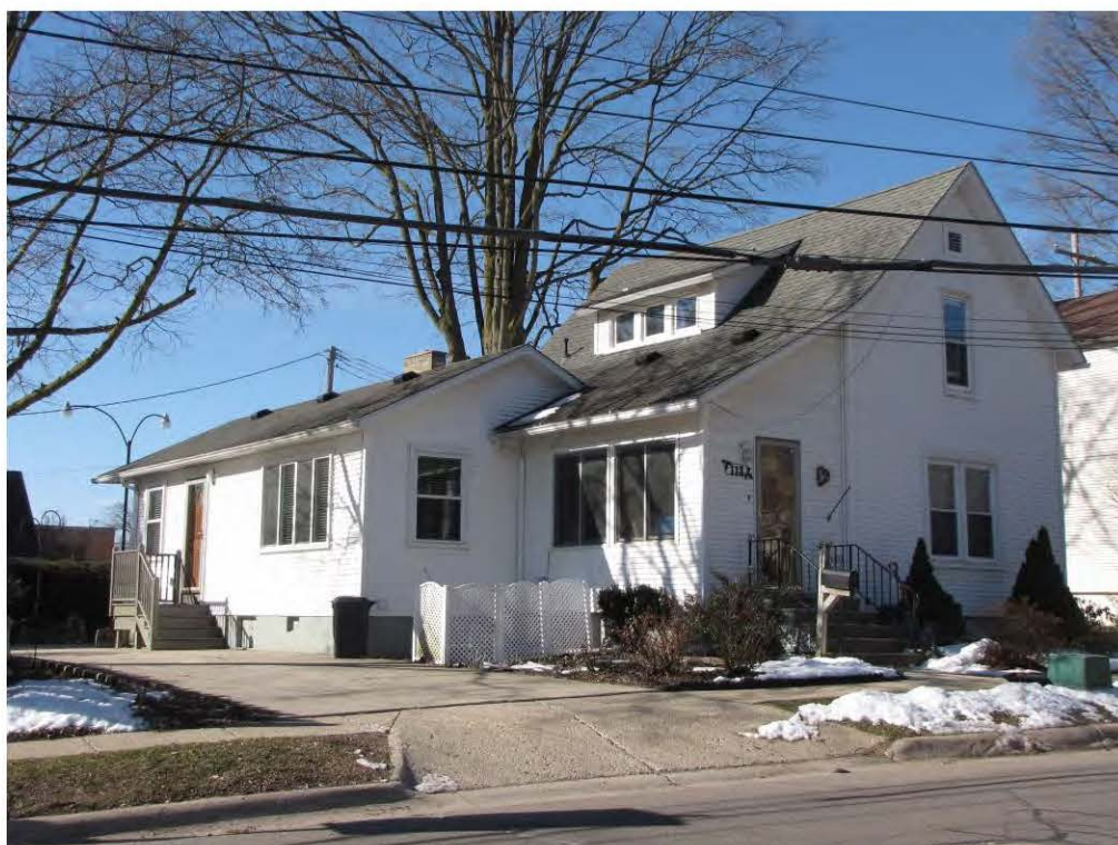
Randolph 113_Looking Southwest
