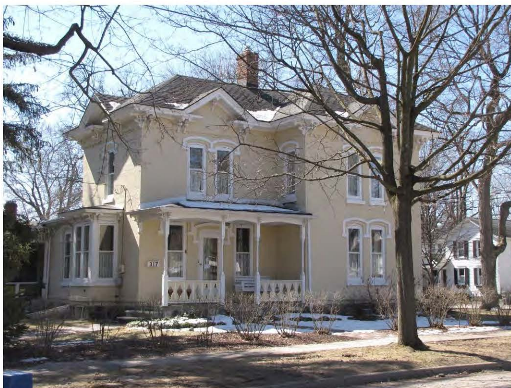
Dunlap West 317_Looking Southwest
