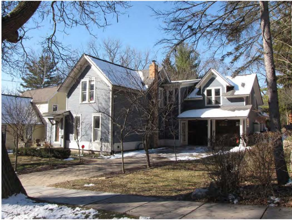
Rogers North 227_Looking Southwest
