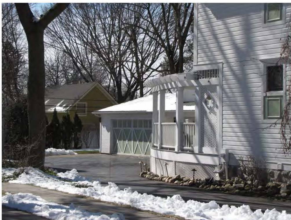
Dunlap West 537, Garage_Looking Southwest
