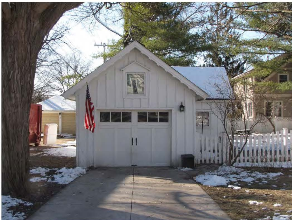
Cady West 521, Carriage House_Looking South
