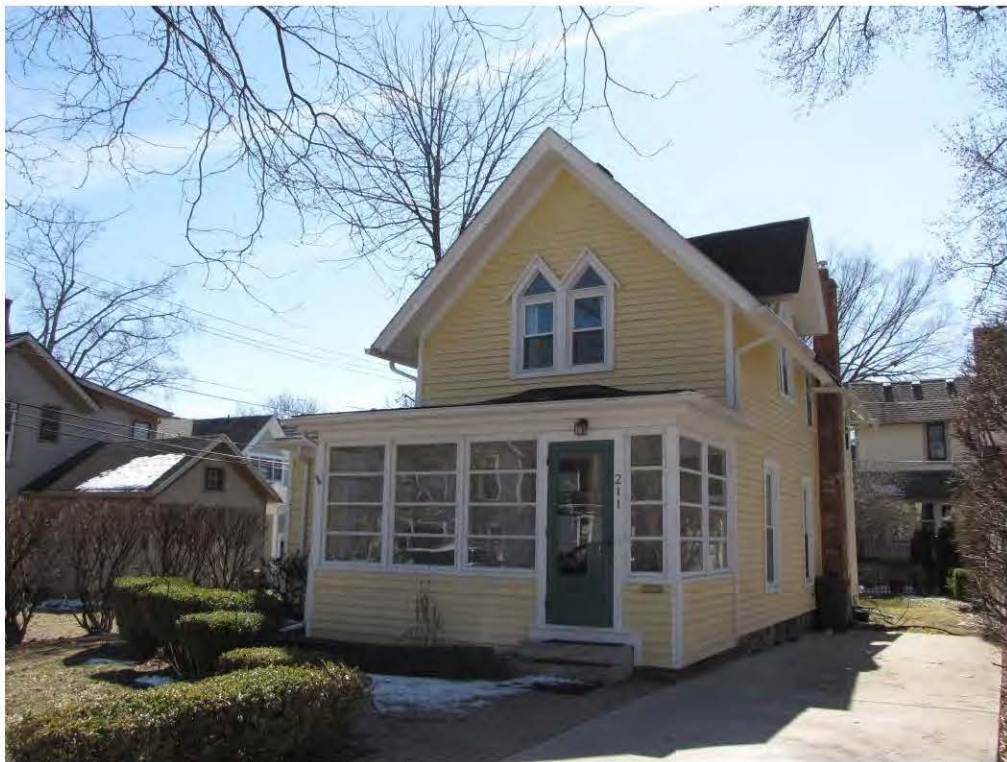
Dunlap West 211_Looking Southeast
