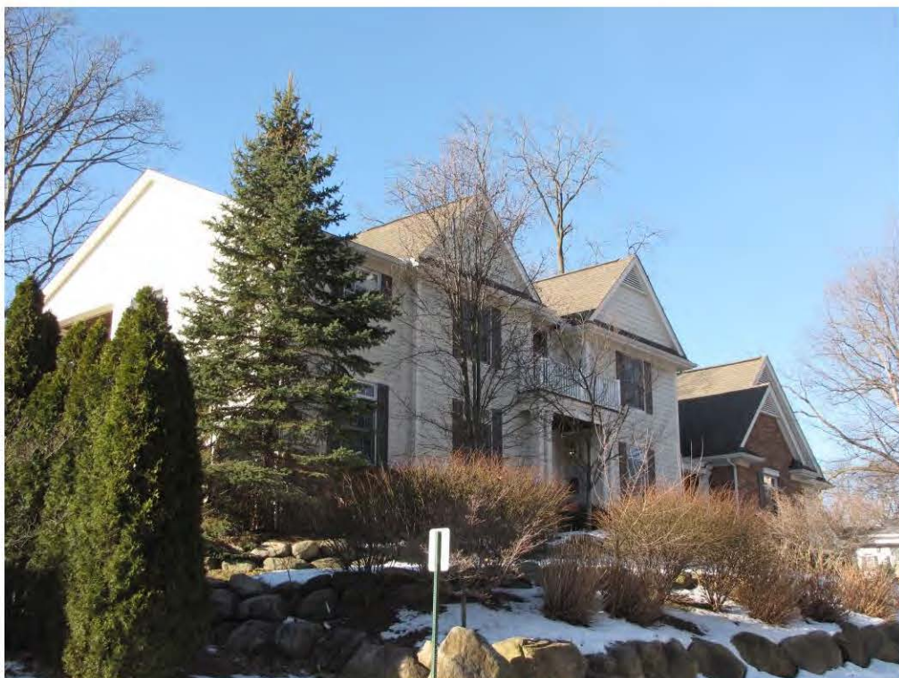
Linden Court 515_Looking Southwest
