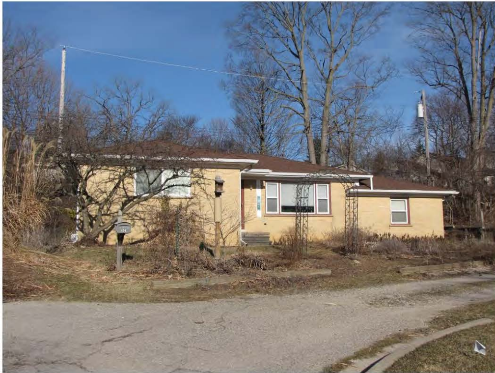
Linden Court 531_ Looking Northwest
