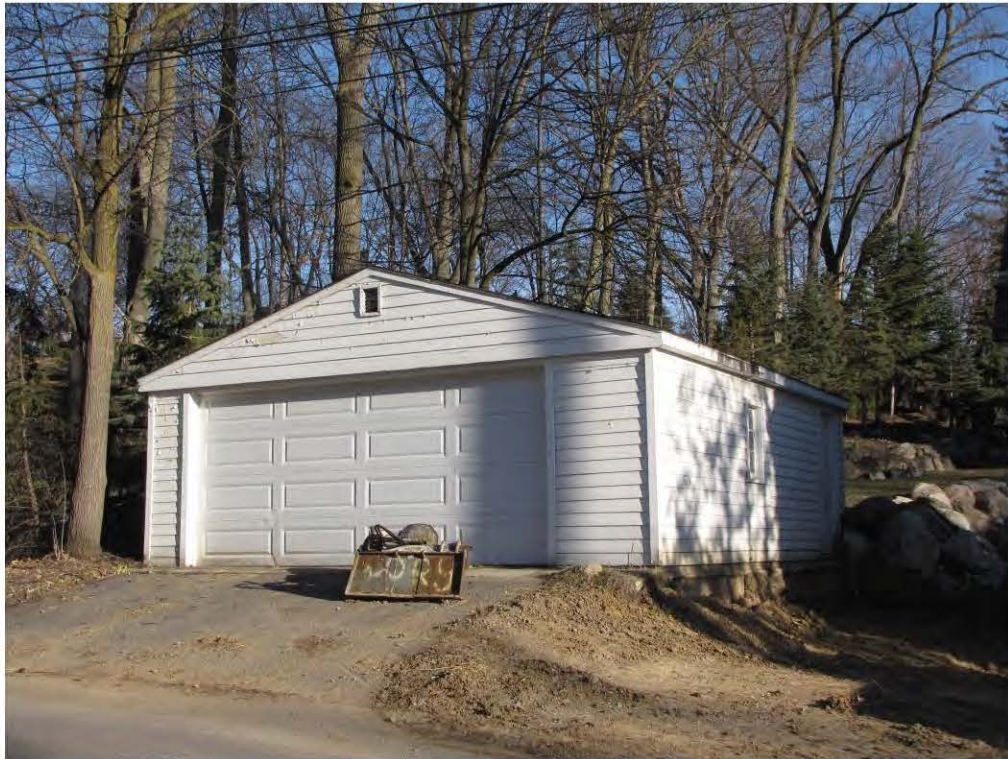
Rogers North 333, Garage_Looking Northwest
