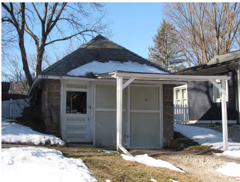
Randolph 509, Garage_Looking South
