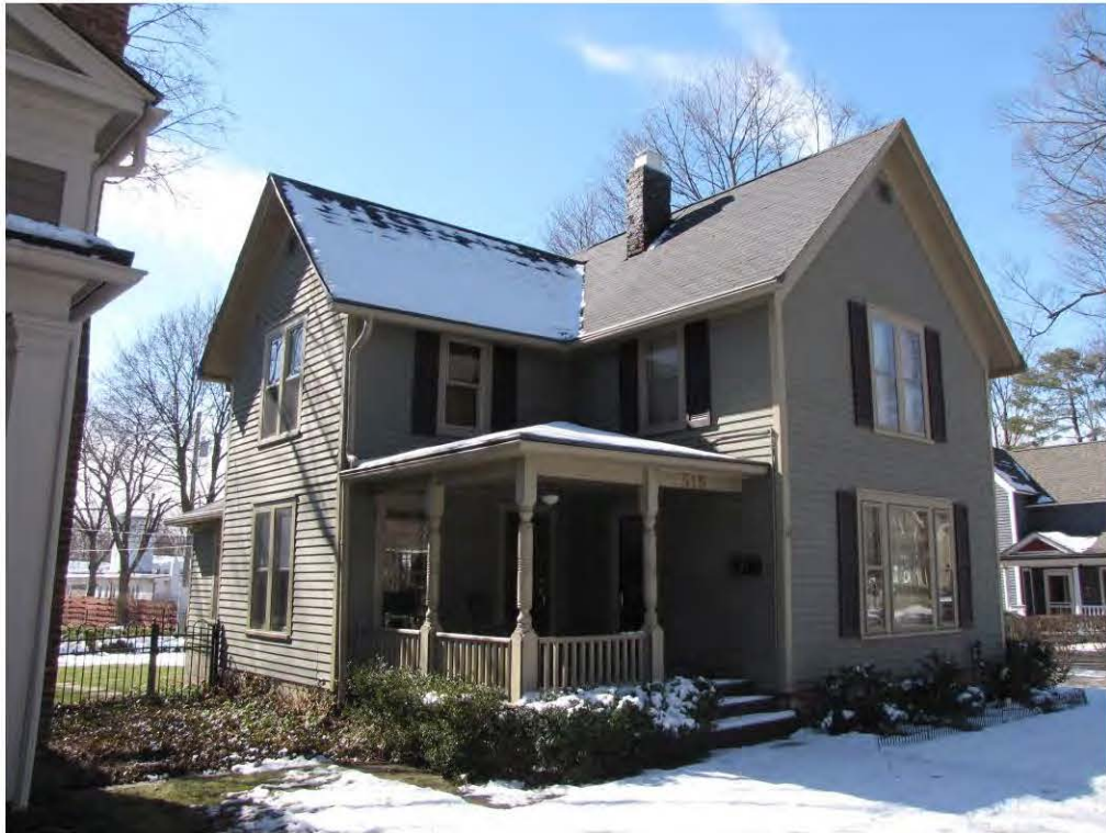
Dunlap West 515_Looking Southwest
