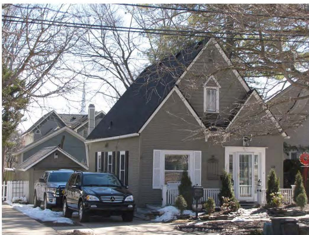
West 228_Looking Southeast
