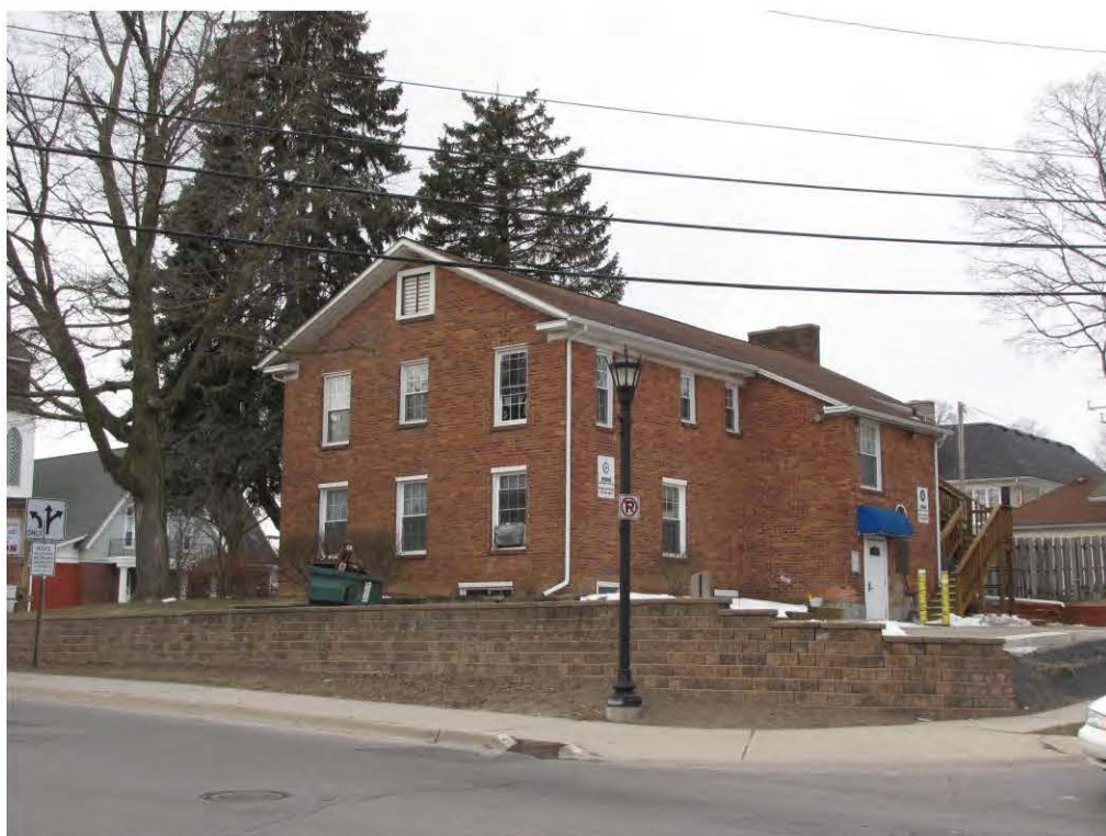
Dunlap West 100_Looking Southwest
