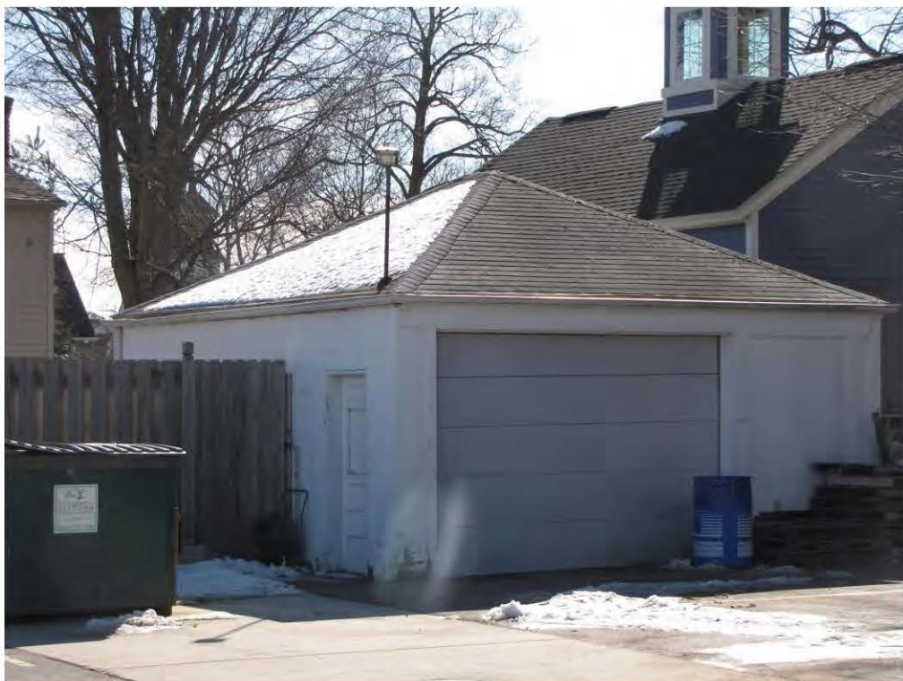
Wing North 217, Garage_Looking Southeast
