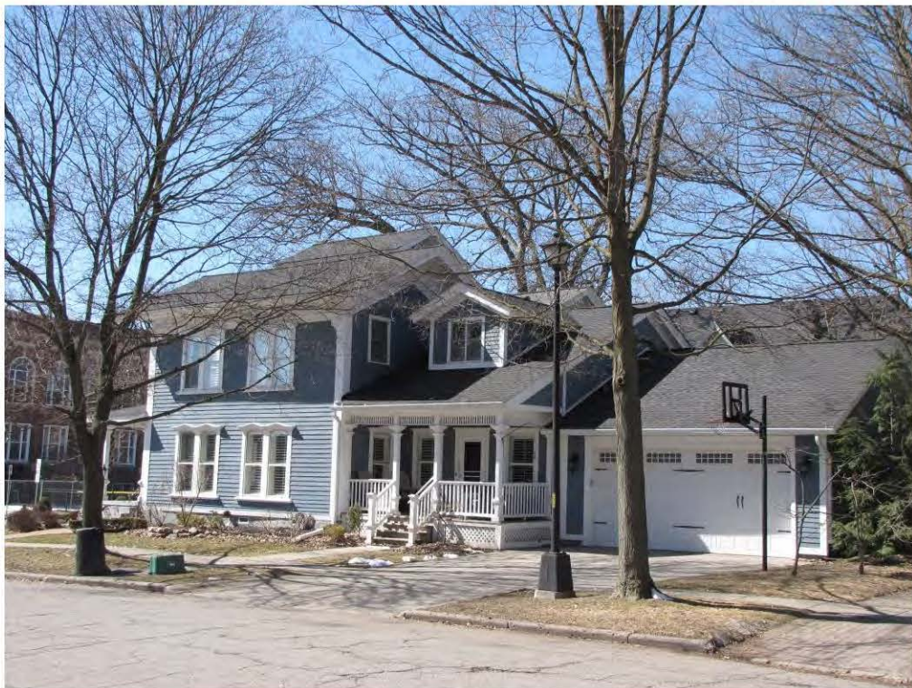
Main West 404_Looking Southwest
