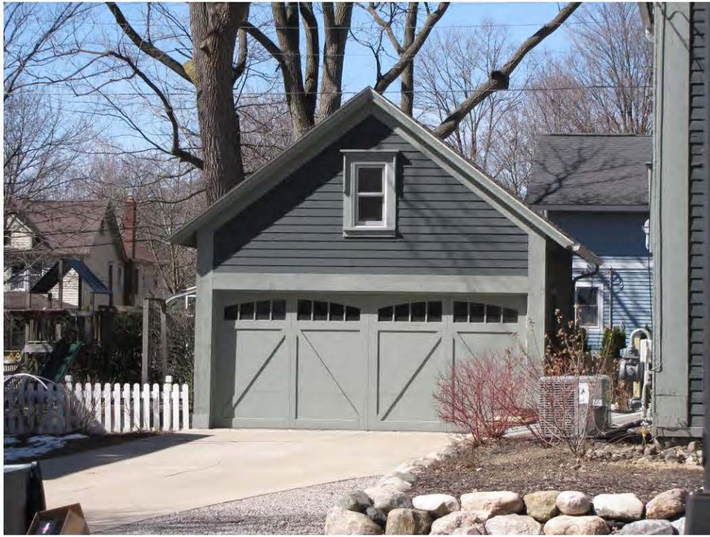
Dunlap West 401, Garage_Looking West
