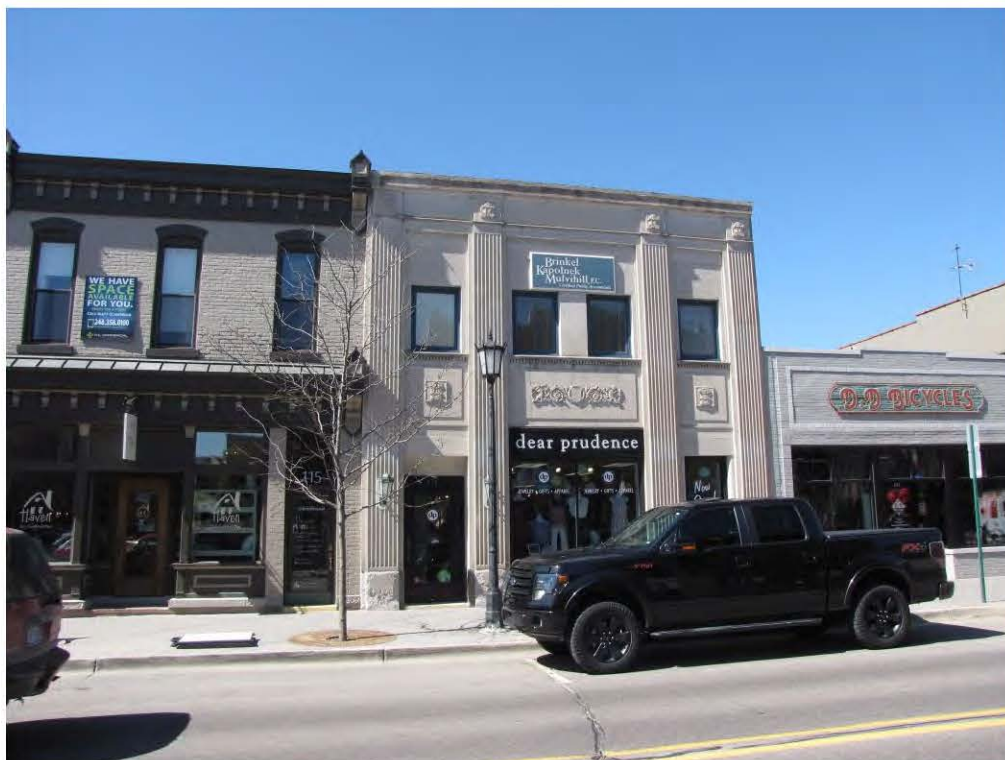
Center North 119_Looking Northeast
