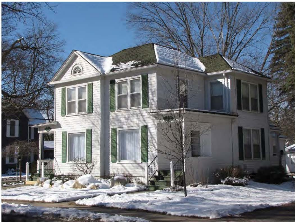
Rogers North 101_Looking Southwest
