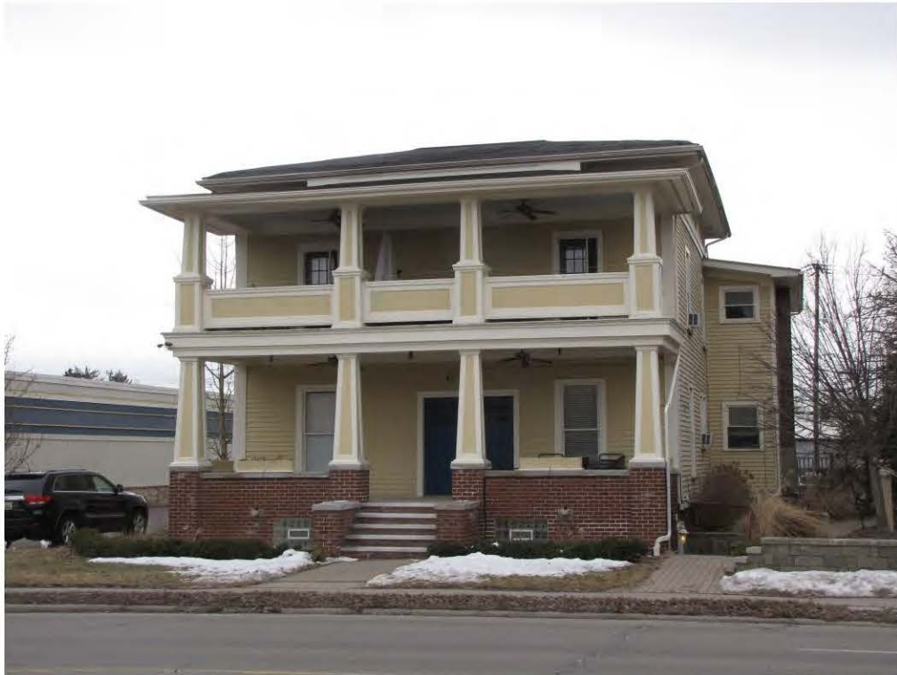
Main East 450_Looking Southeast
