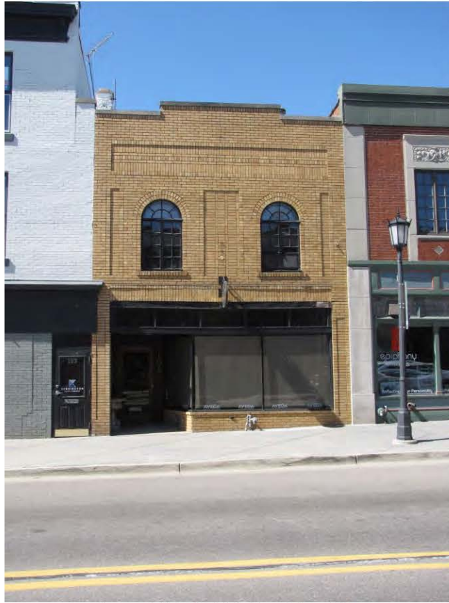
Center North 105_Looking West
