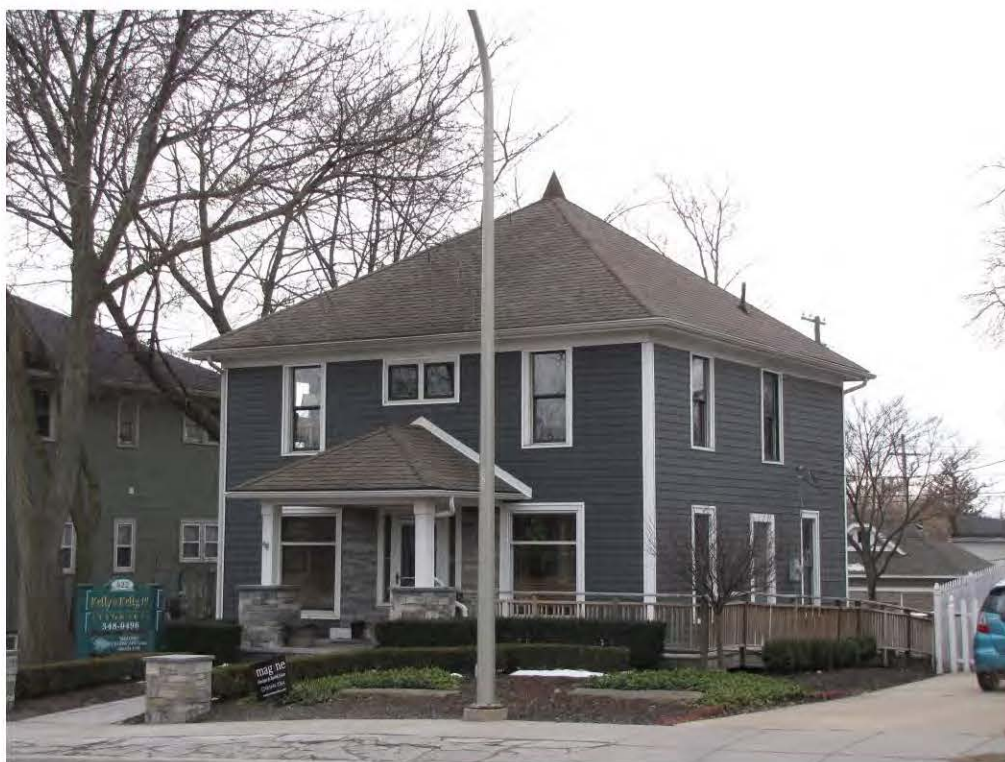
Main East 422_Looking Southeast
