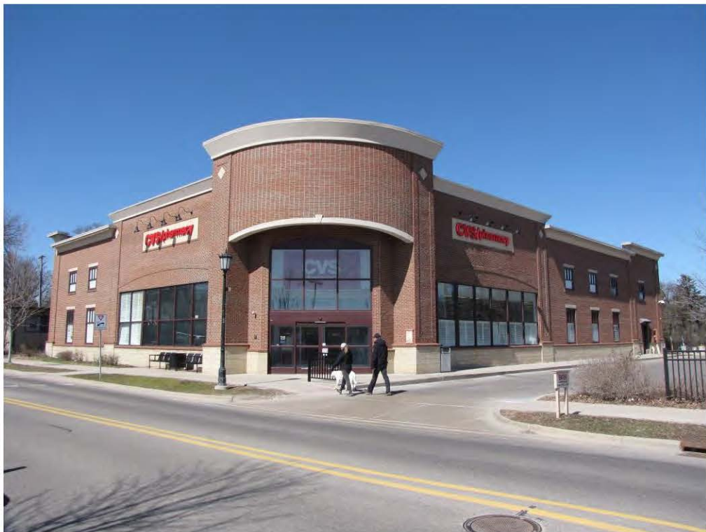
Dunlap East 133_Looking Northwest
