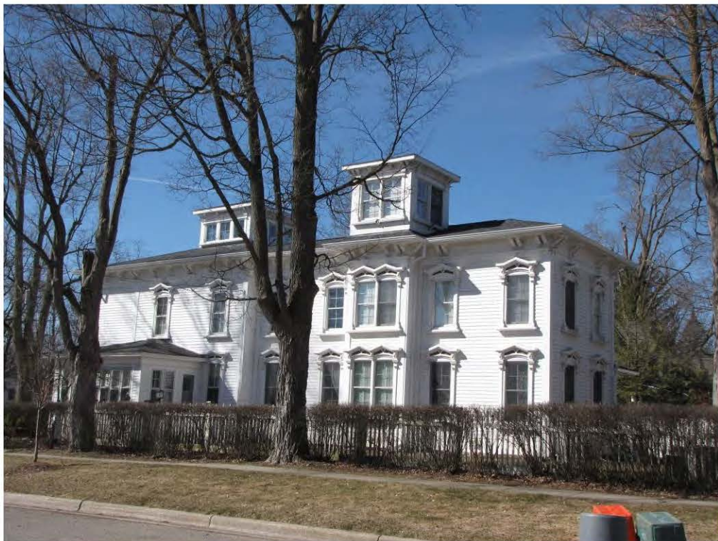
Dunlap West 404_Looking Southwest
