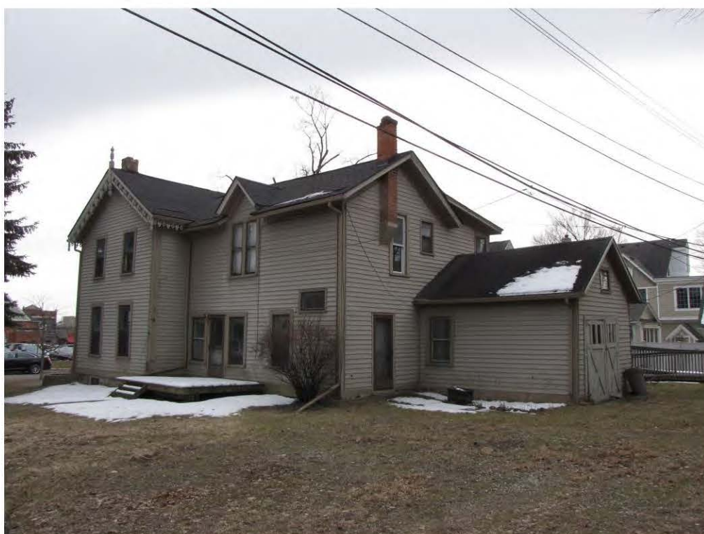
Wing North 129_Looking Southeast
