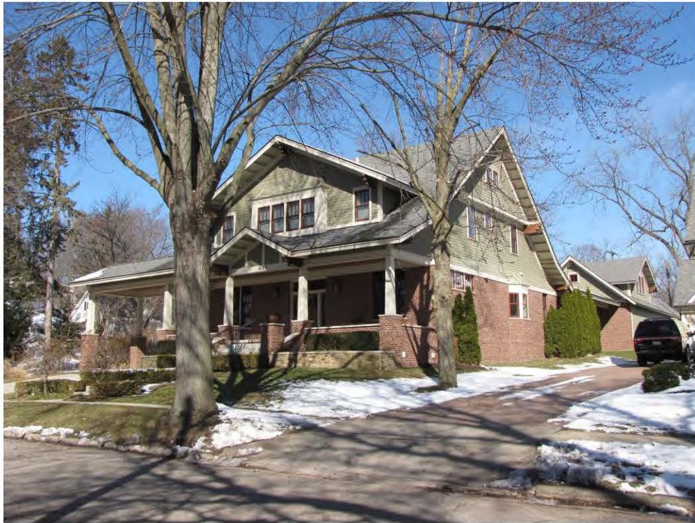
Dubuar 430_ Looking Northwest
