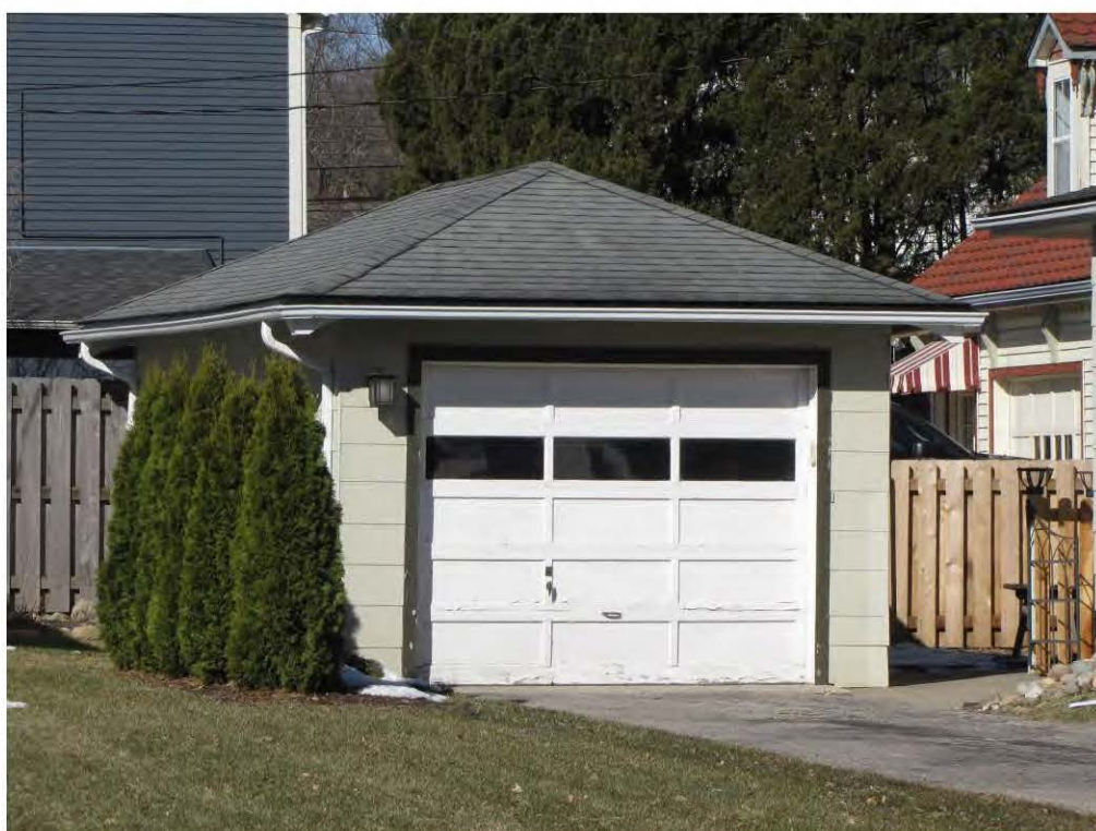
High 213, Garage_Looking West
