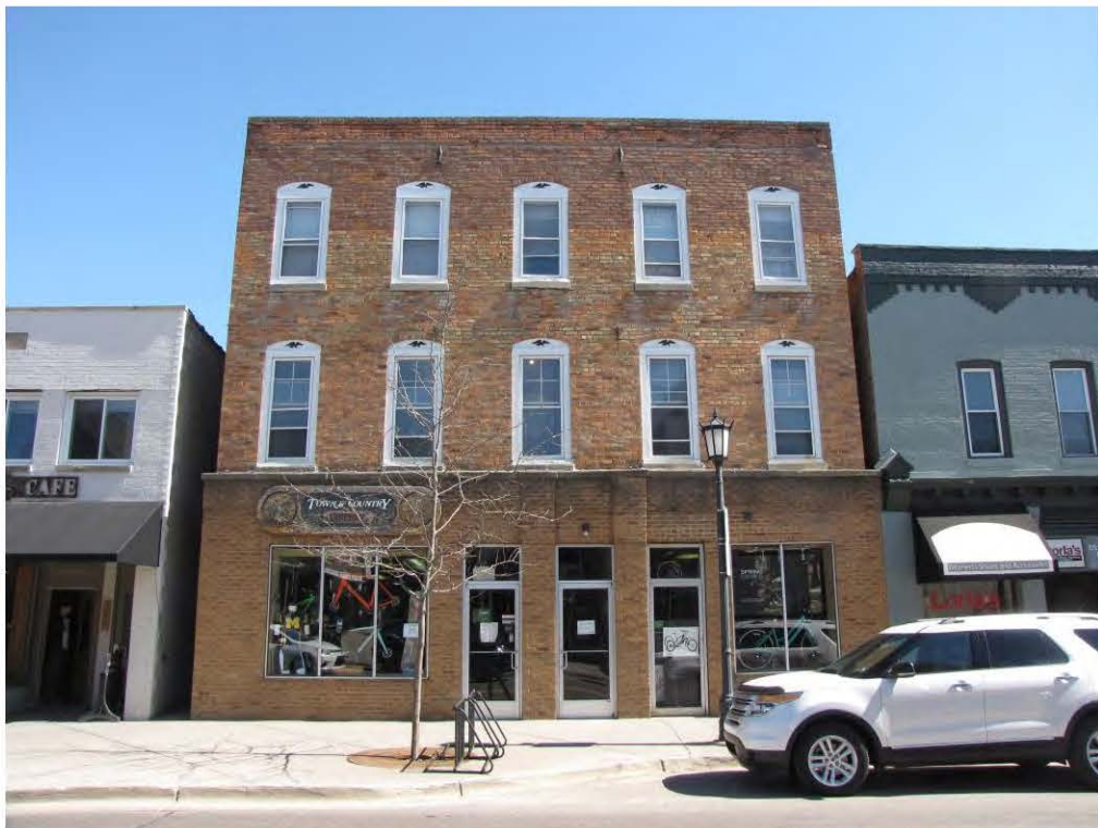
Center North 144-148_ Looking East
