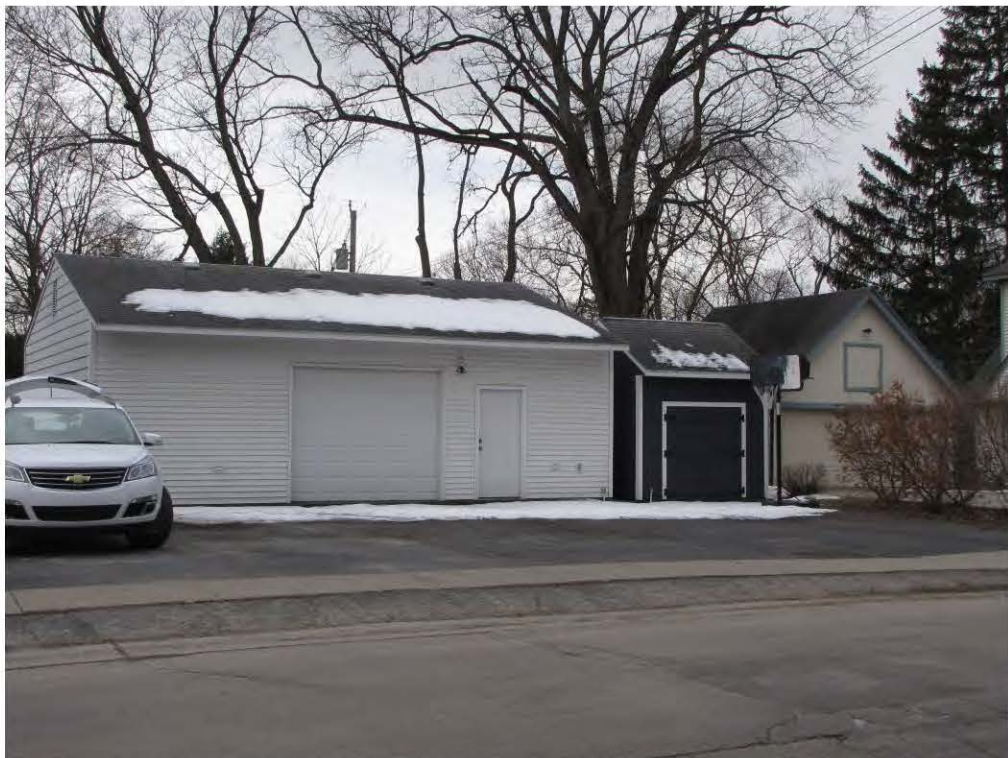
Rogers South 102, Garage_Looking Southwest
