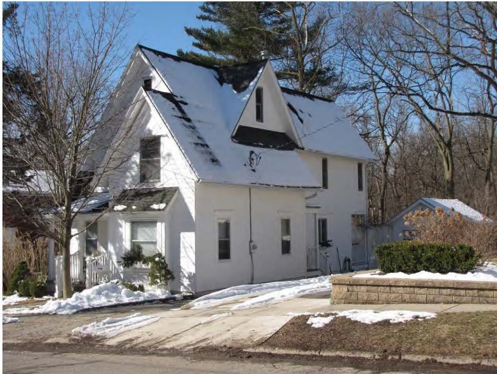
Rogers North 207_Looking Southwest
