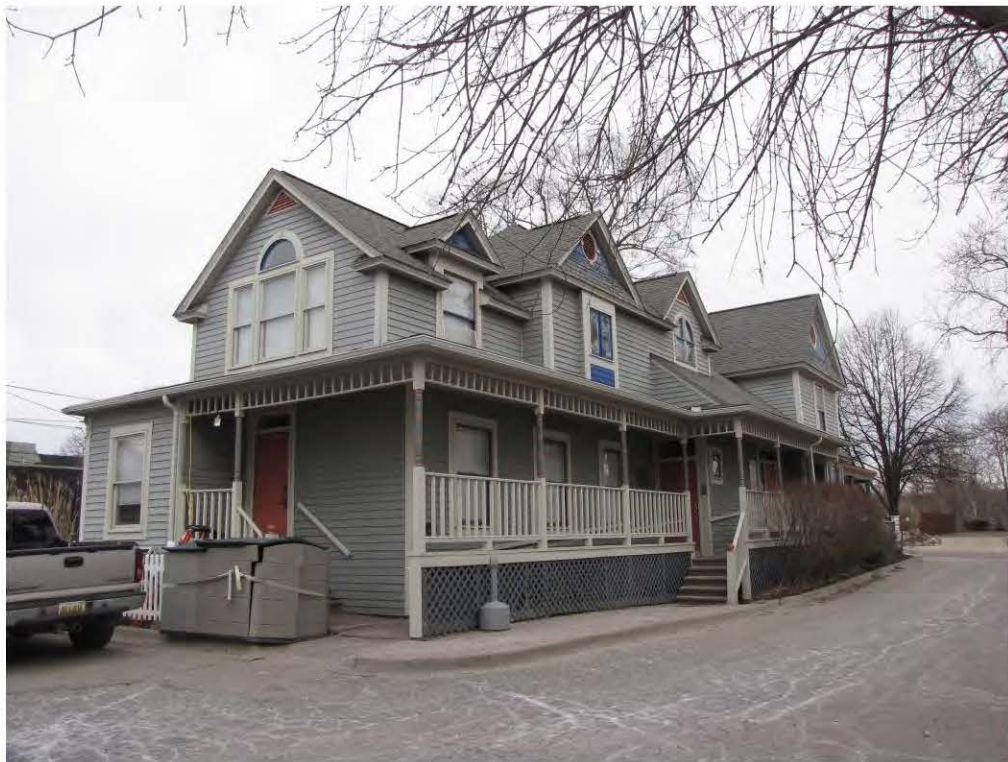
Main East 332_Looking Northwest
