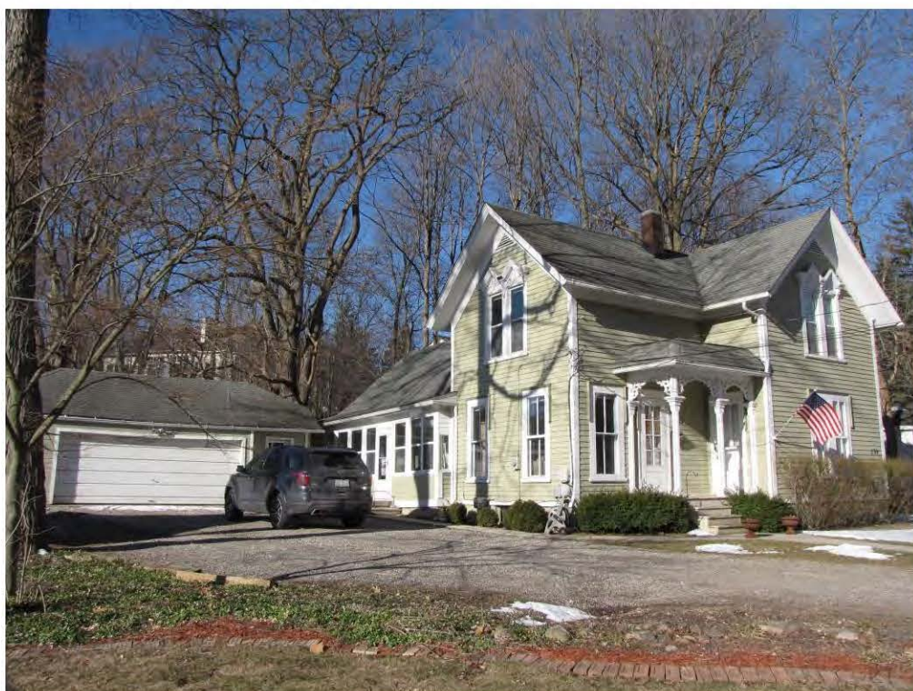
Randolph 537-539_Looking Southwest
