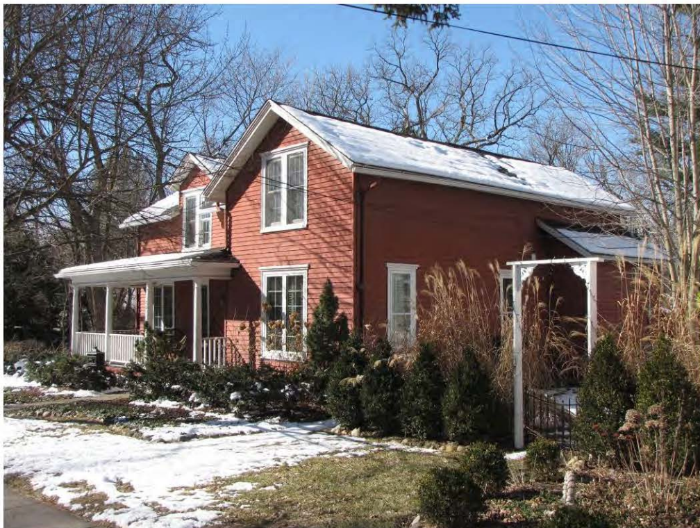
Rogers North 201_Looking Southwest
