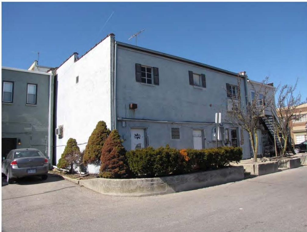
Center North 150_Looking Northwest
