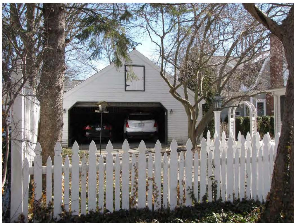
Main West 548, Garage_Looking East
