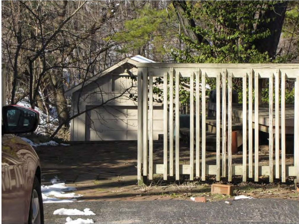
Randolph North 117, Garage_Looking West
