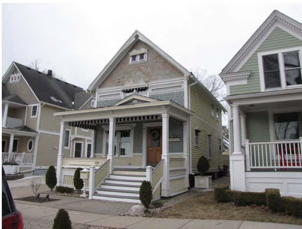
Wing North 121_Looking Southwest
