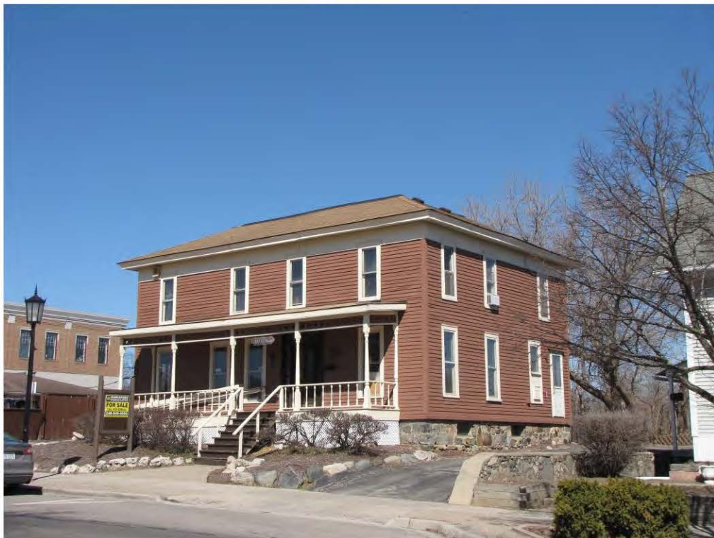
Main East 341_Looking Northwest
