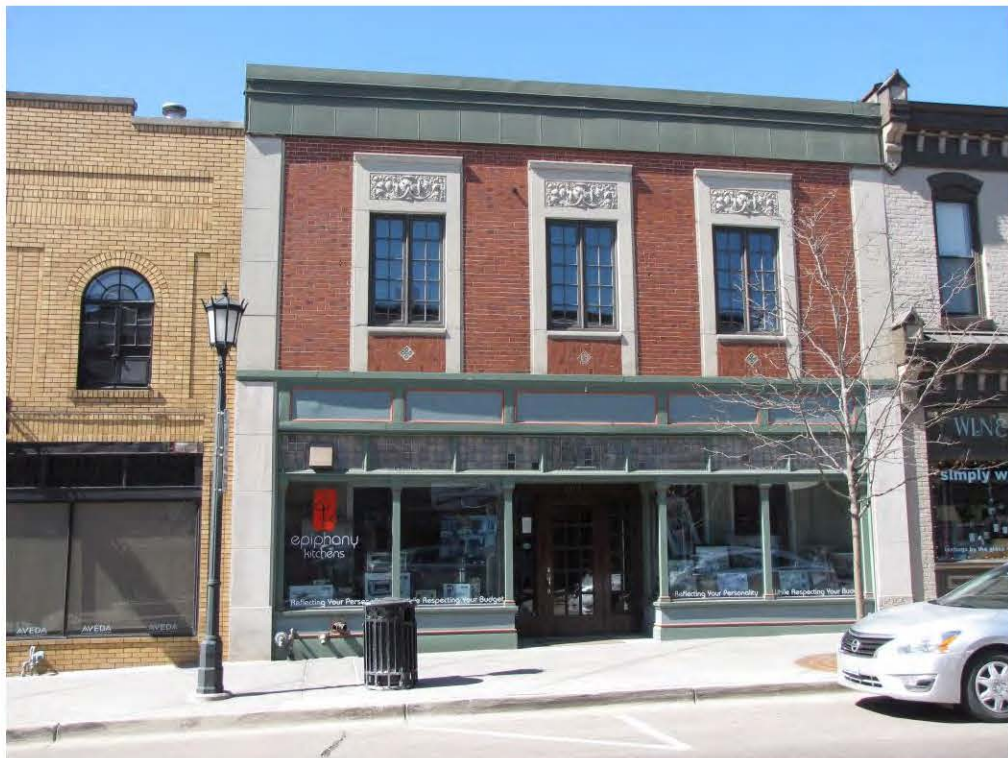
Center North 107_Looking West
