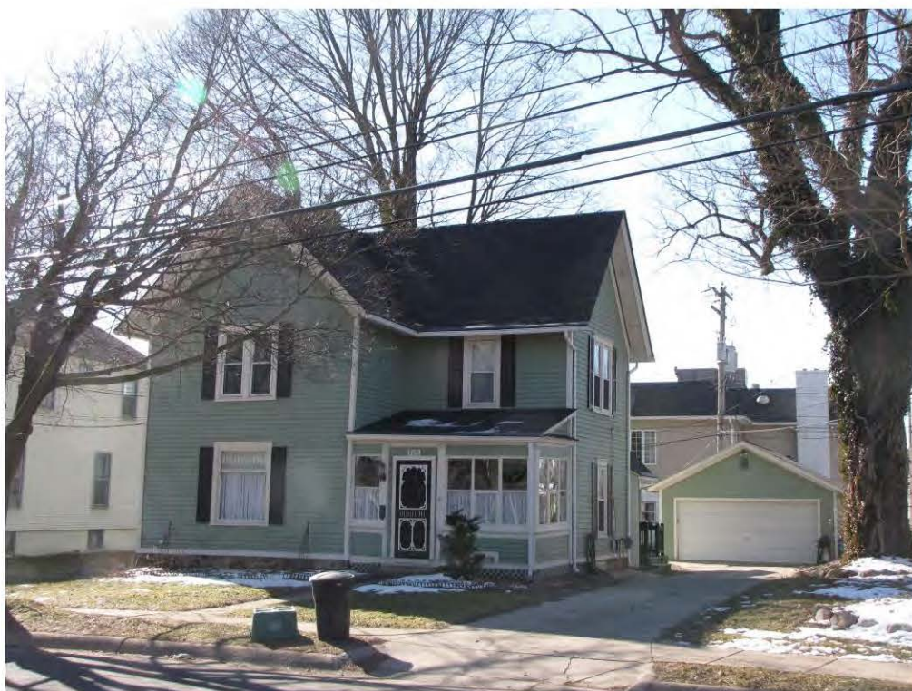
Randolph 125, Garage_Looking South
