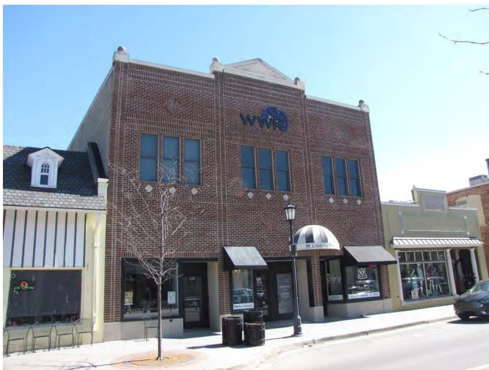
Center North 124-128_Looking Northeast
