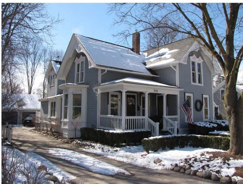
Main West 521_Looking Southwest
