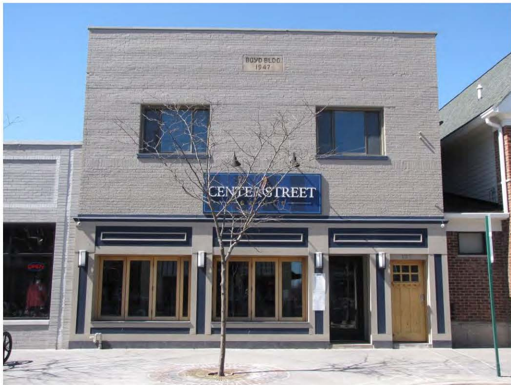
Center North 135-137_Looking West
