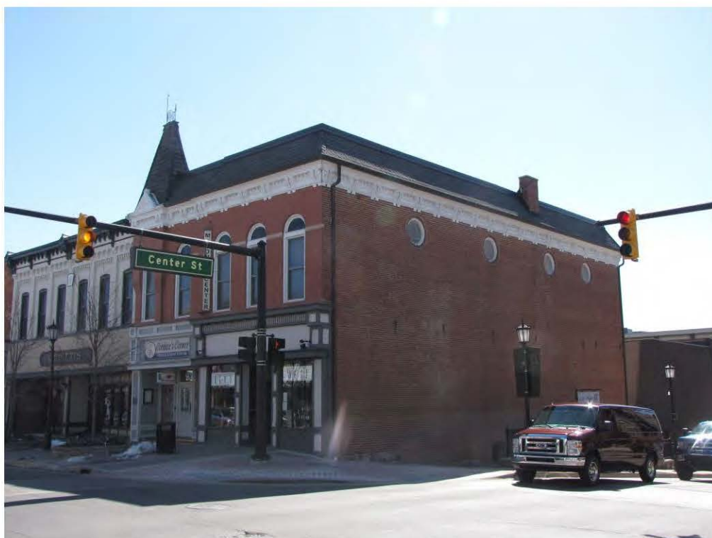
Main East 102-106 and Center South 113 Looking Southeast
