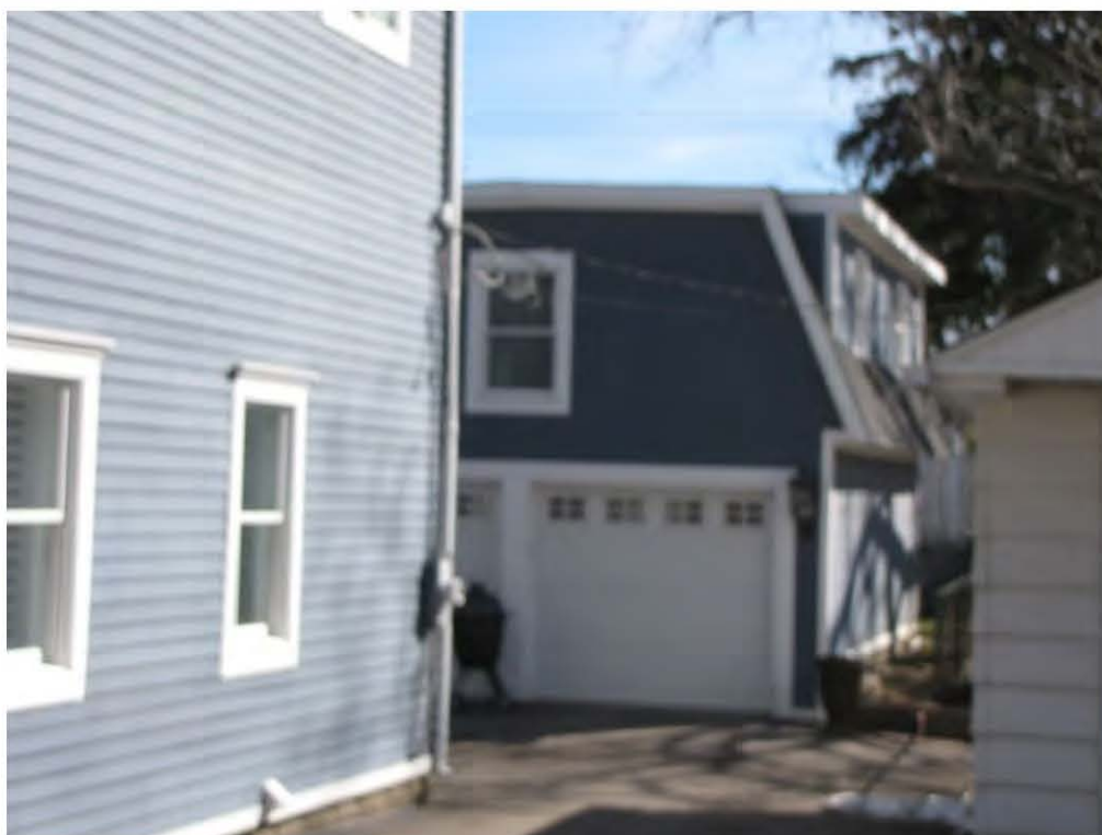
Linden 254, Garage_Looking East
