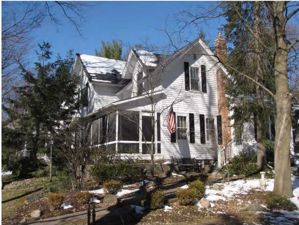
Dubuar 440_ Looking Northwest
