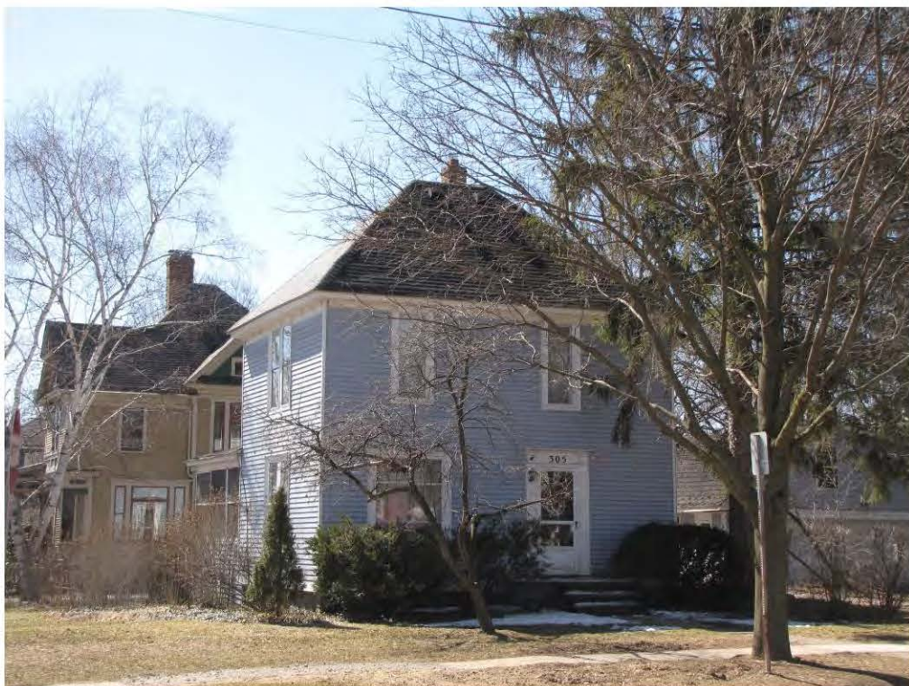
Dunlap West 305_Looking Southwest
