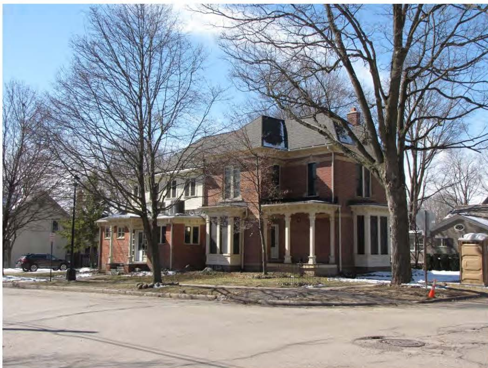
Dunlap West 501_Looking Southwest
