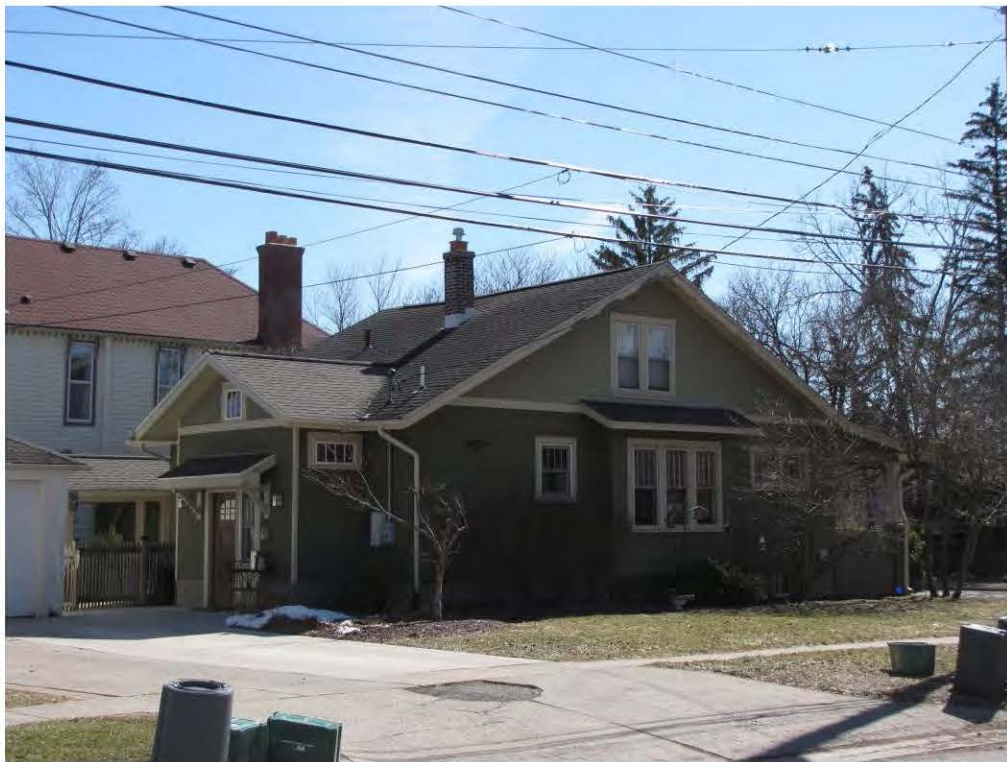
Dunlap West 314_Looking Southeast
