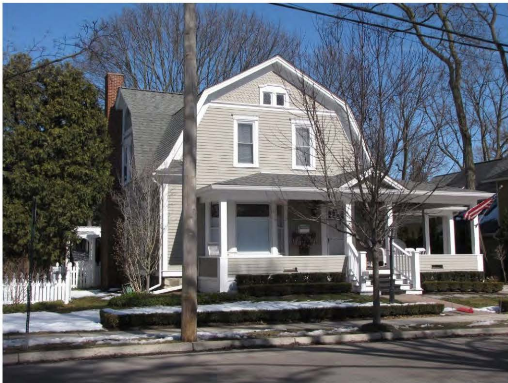
Main West 542_Looking North
