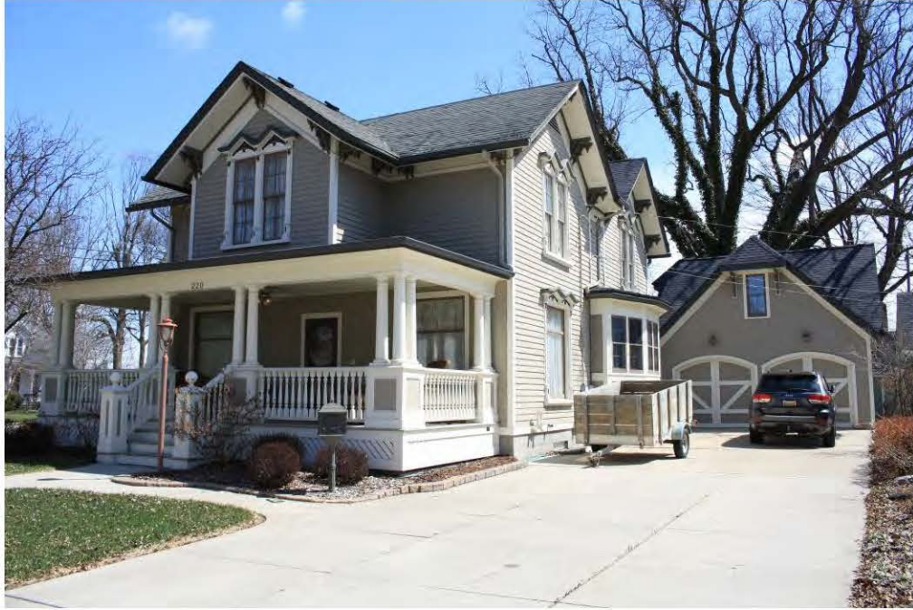
Wing North 220_Looking Southwest
