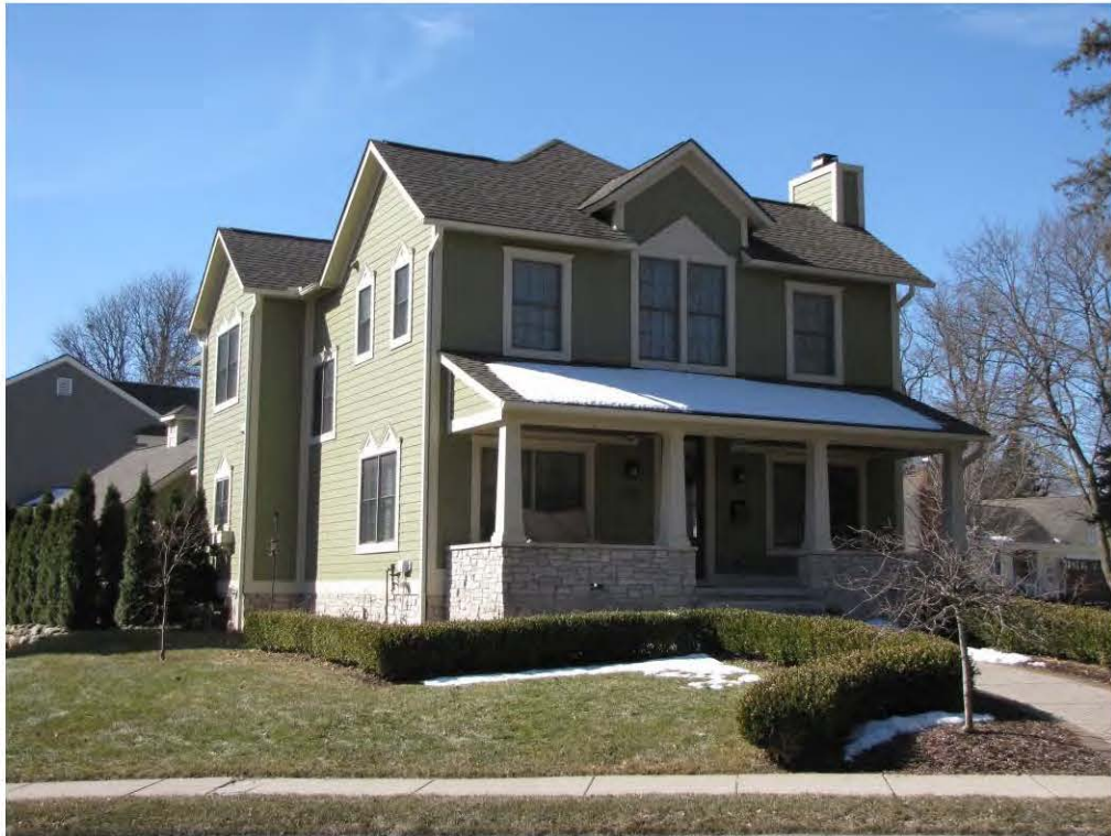
Randolph 413_Looking Southwest
