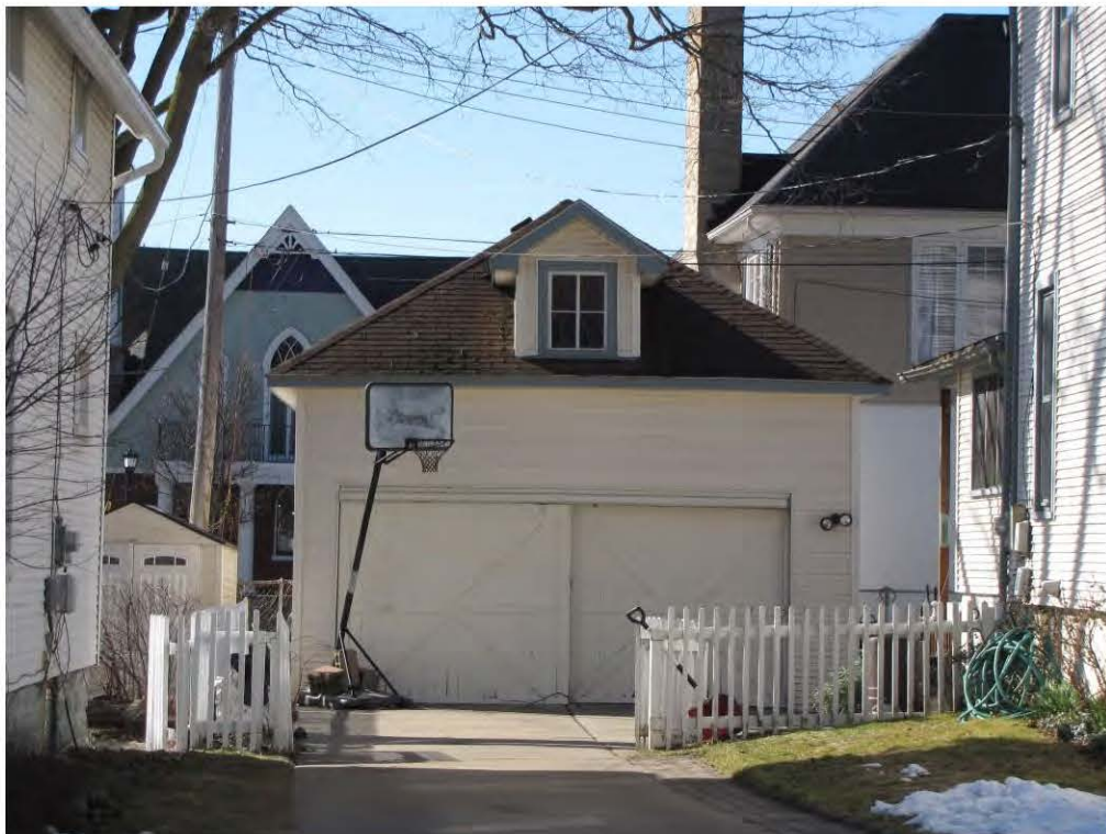
Randolph 119, Garage_Looking South
