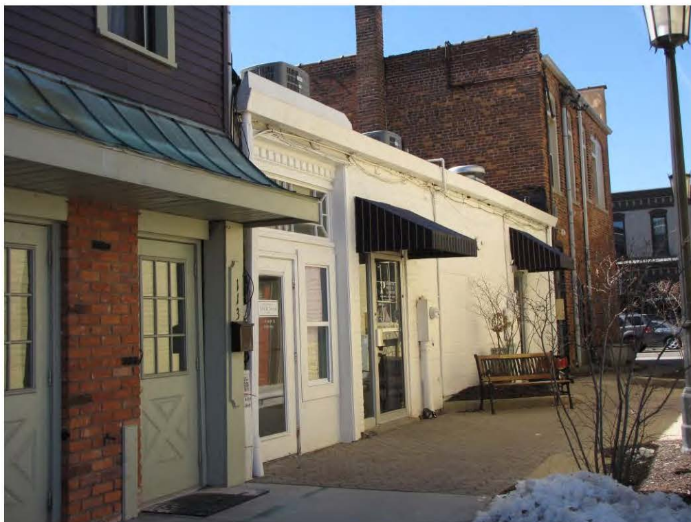
Main East 103-107_Looking North
