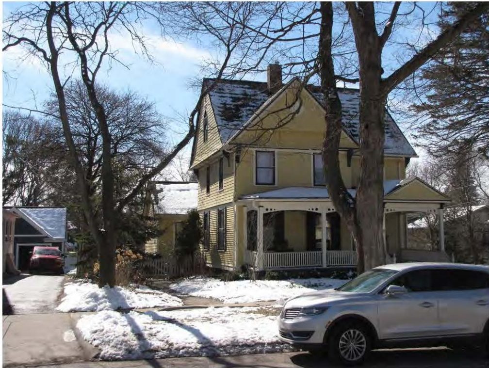
Dunlap West 549_Looking Southwest
