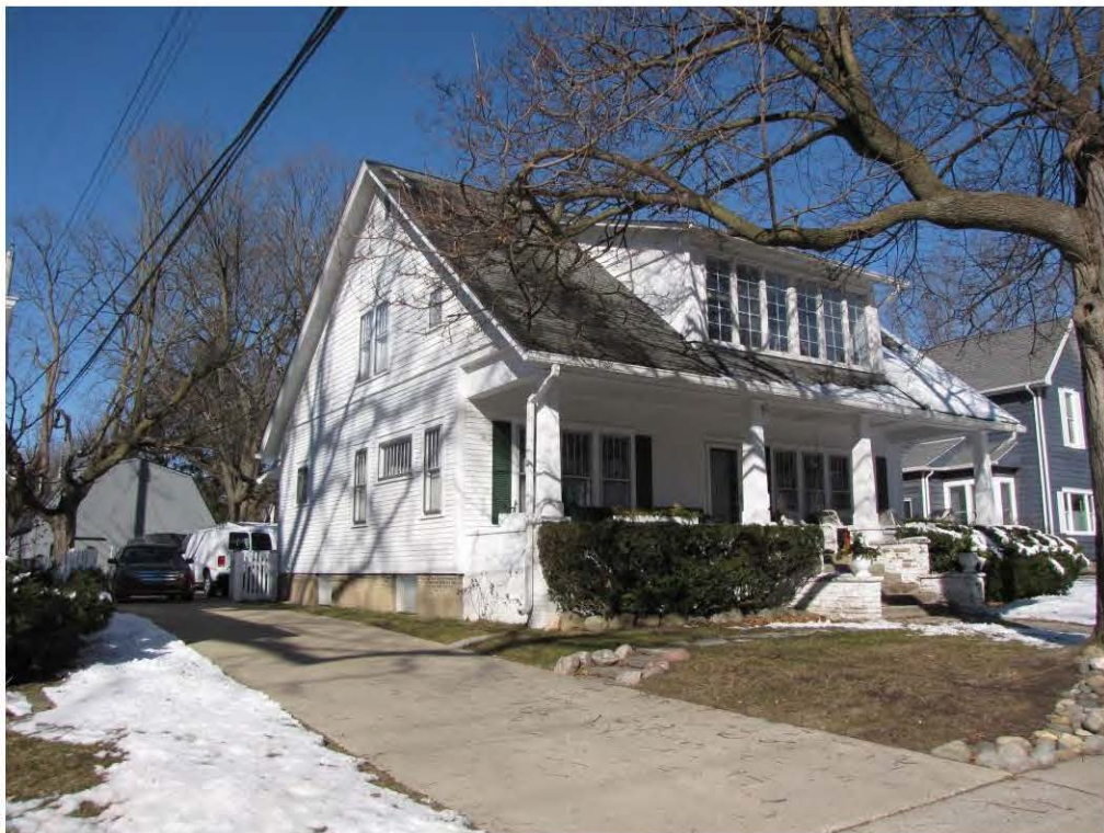
Rogers South 110_Looking Northwest
