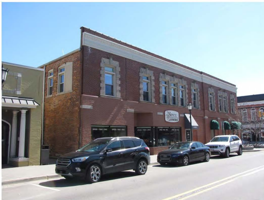
Main East 101 and Center North 108-110 Looking Southeast
