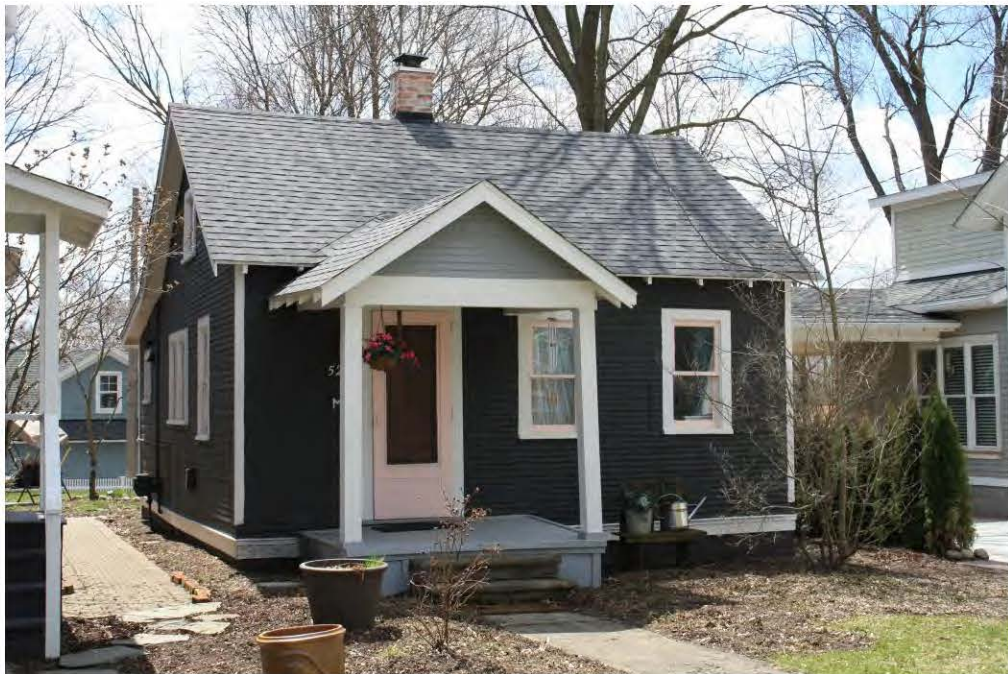
Main West 523_Looking Southwest
