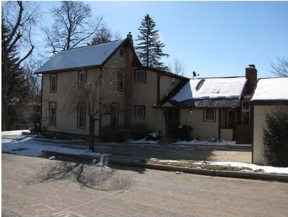
Rogers North 231_Looking Southwest
