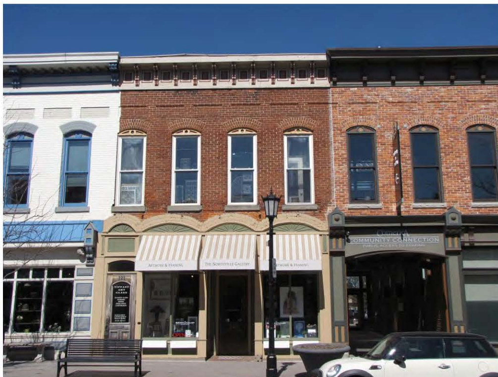
Main East 121-123_Looking North
