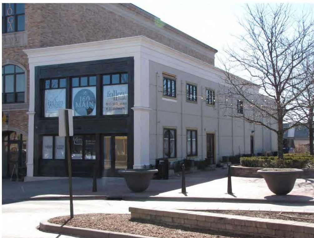
Main East 160_Looking Southeast
