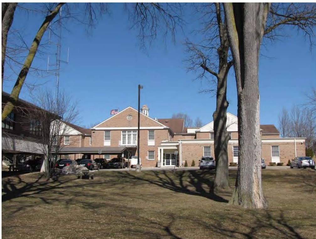
Main West 215_Looking North
