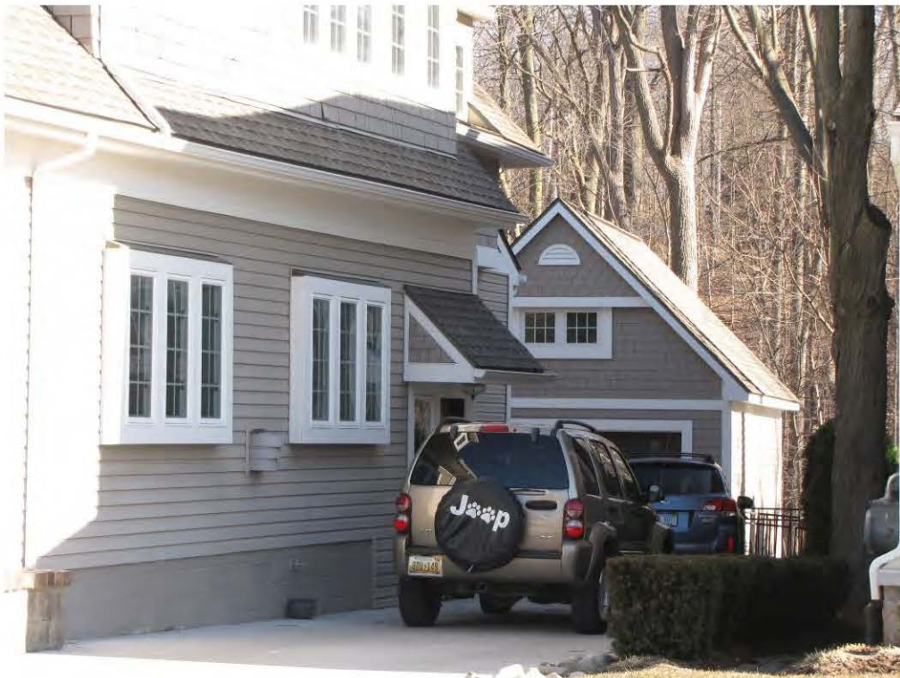
Randolph 418, Garage_Looking North
