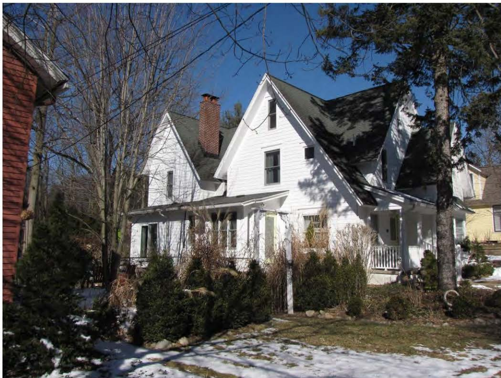
Rogers North 207_Looking Northwest
