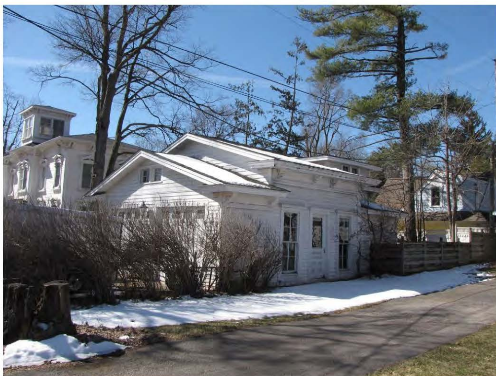
Dunlap West 404, Garage_Looking Southwest
