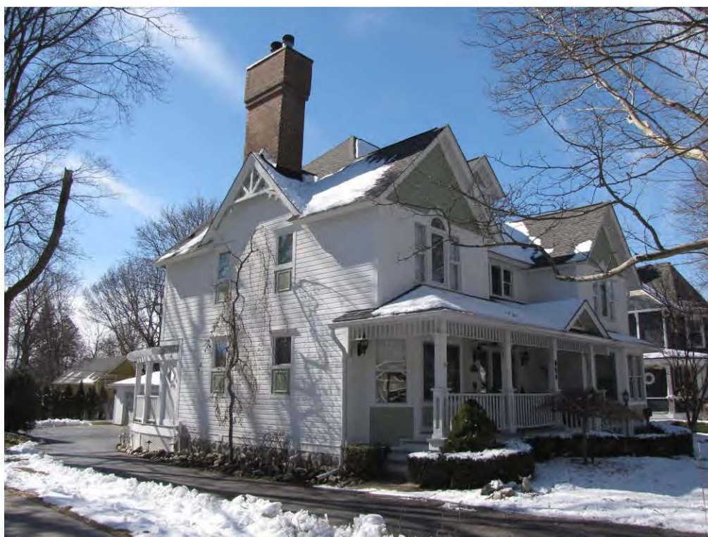
Dunlap West 537_Looking Southwest
