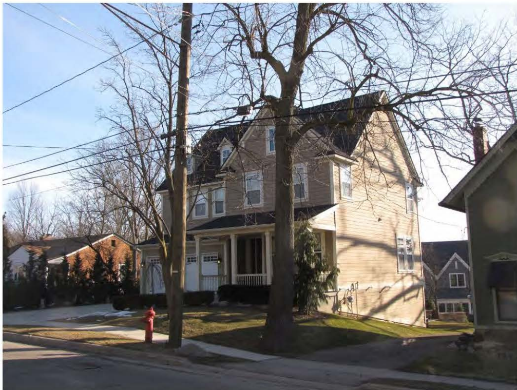
Rogers North 350_Looking Northeast
