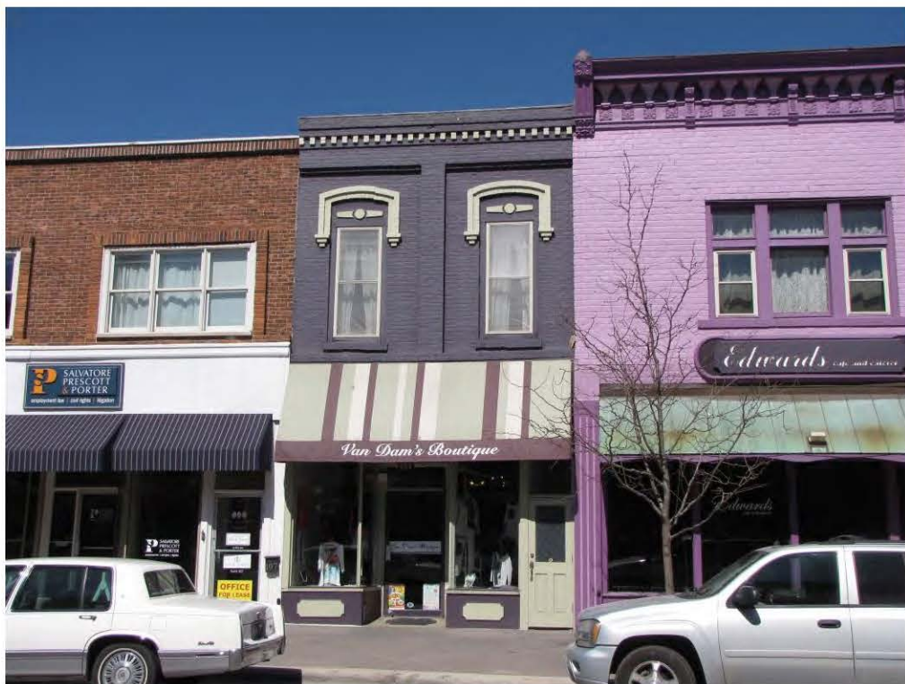
Main East 111_Looking North
