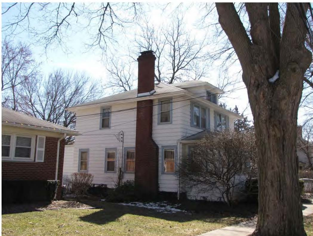
West 114_Looking Southeast
