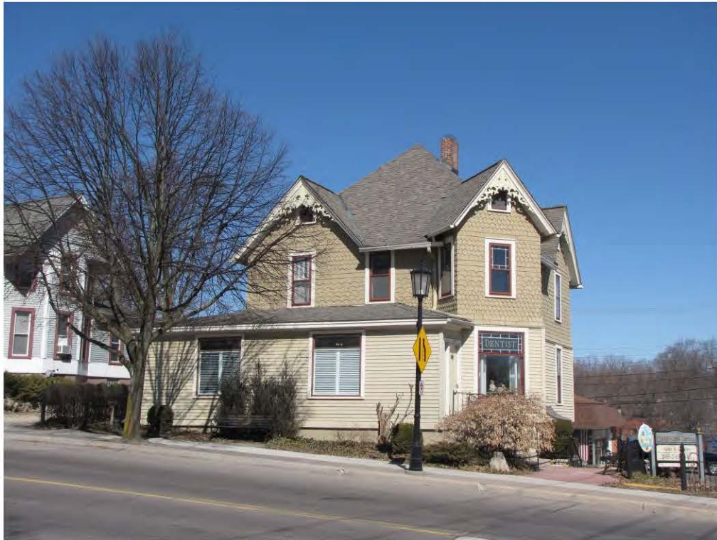
Main East 371_Looking Northwest
