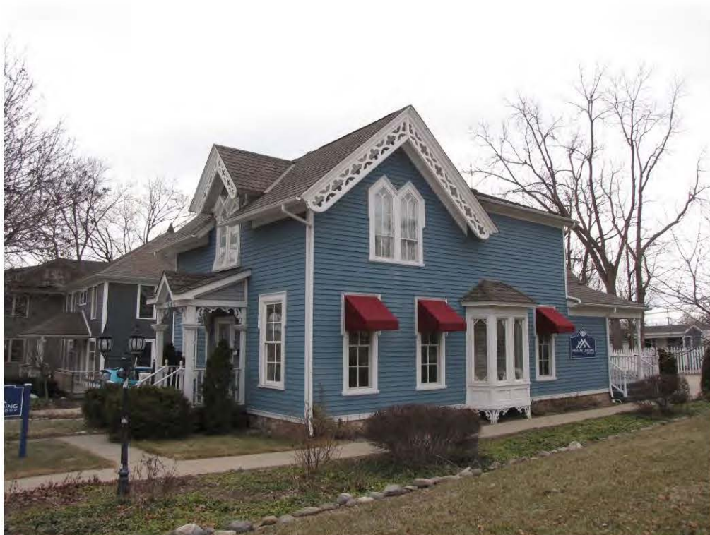
Main East 410_Looking Southeast
