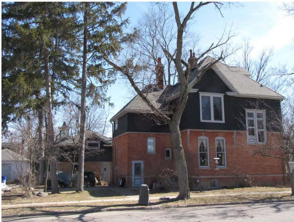
Dunlap West 218_Looking Southeast
