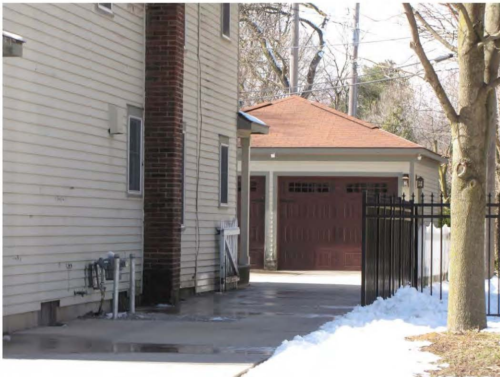
Linden 115, Garage_Looking West
