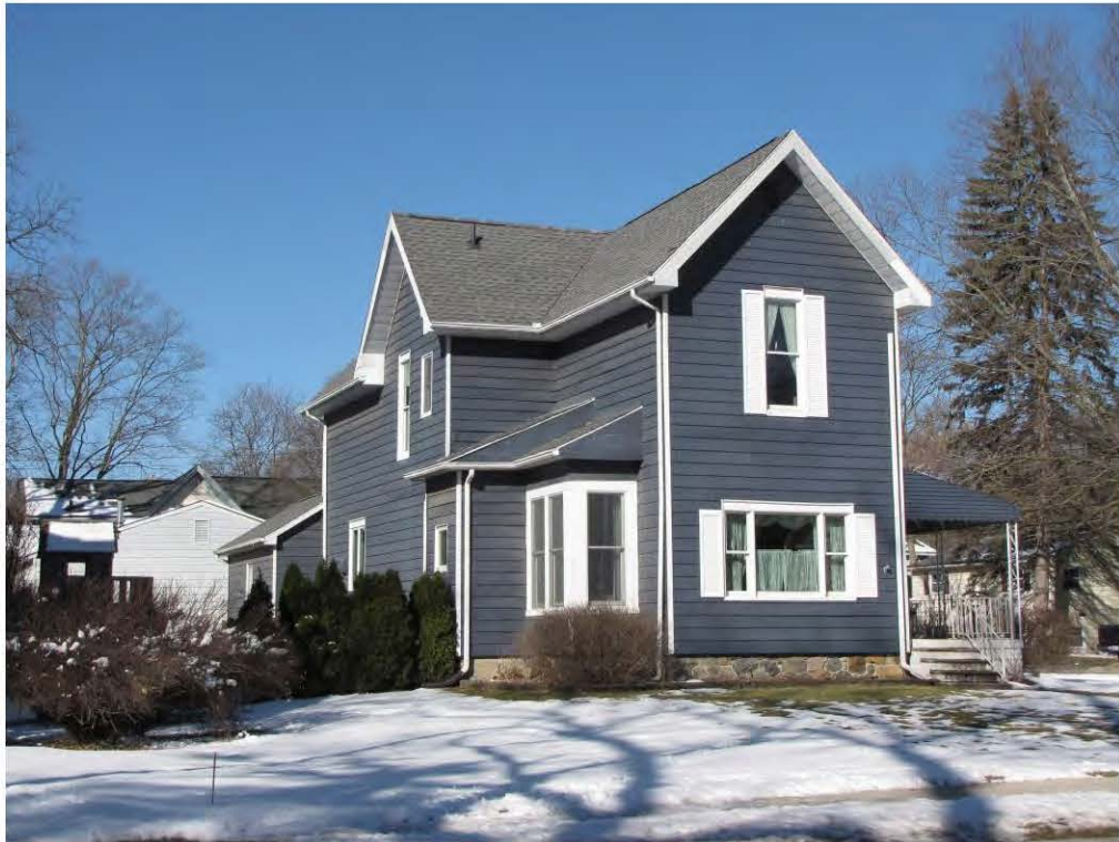
Rogers South 102_Looking Northwest
