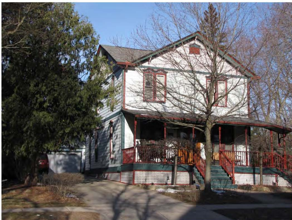
Rogers North 365_Looking Northwest
