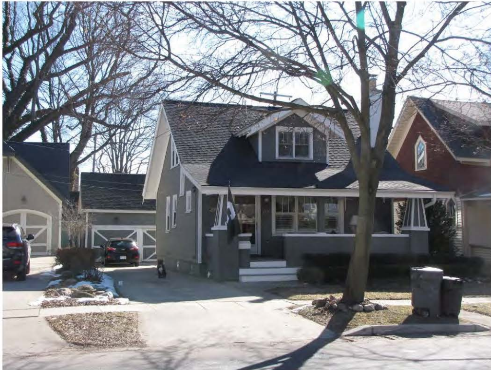
Wing North 214_Looking Southeast
