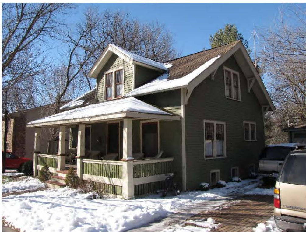
Rogers North 131_Looking Southwest
