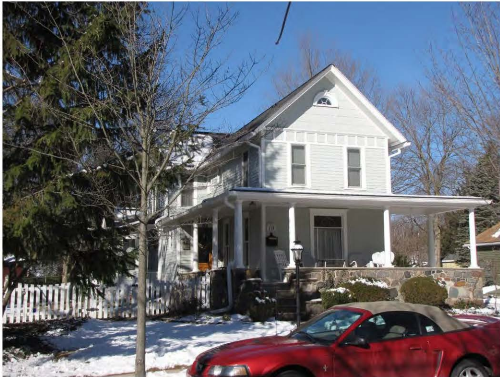
Rogers South 128_Looking Northwest
