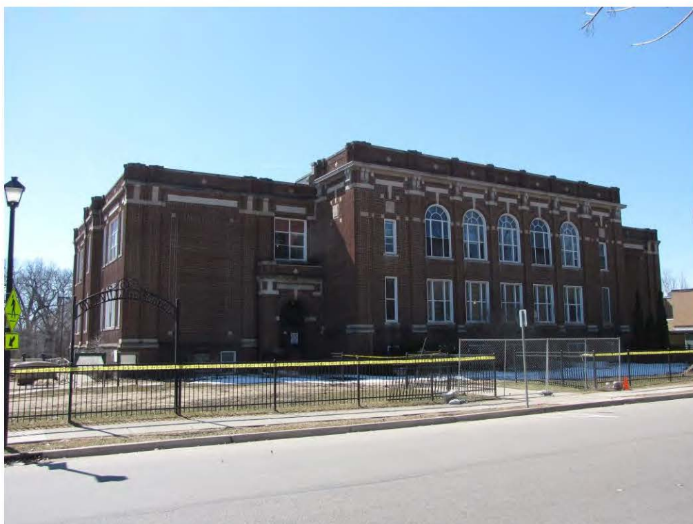
Main West 411_Looking South
