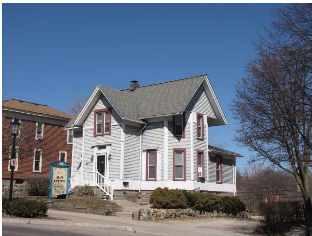
Main East 355_Looking Northwest
