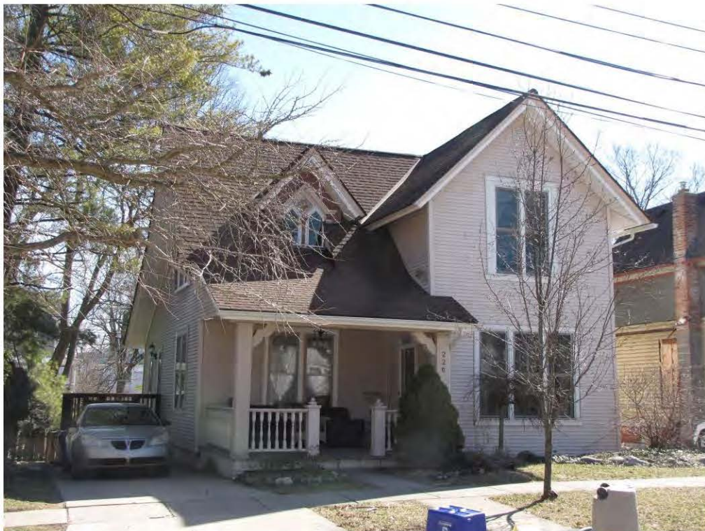
West 226_Looking Southeast
