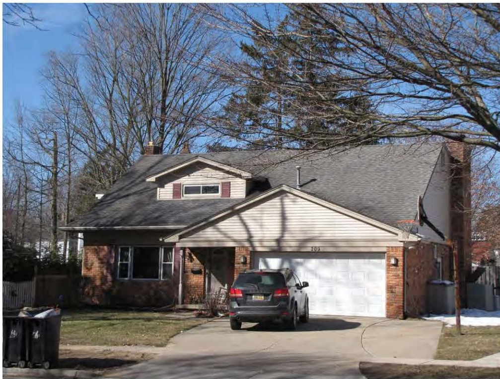
Wing North 209_Looking Southwest
