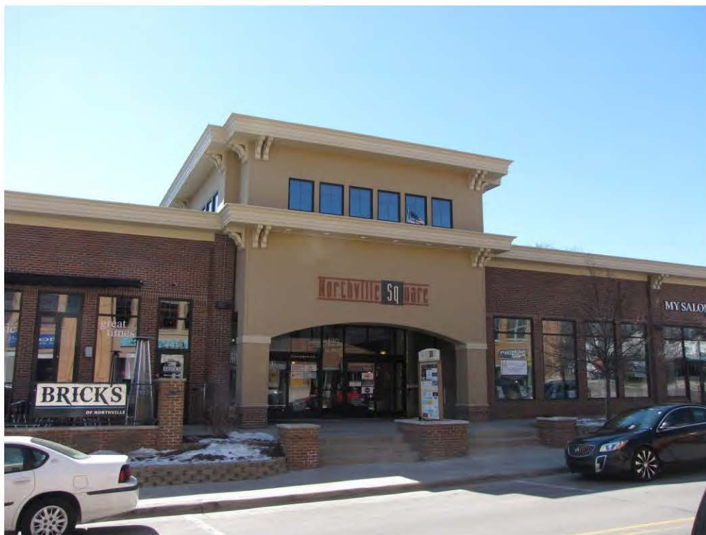
Main West 133_Looking South
