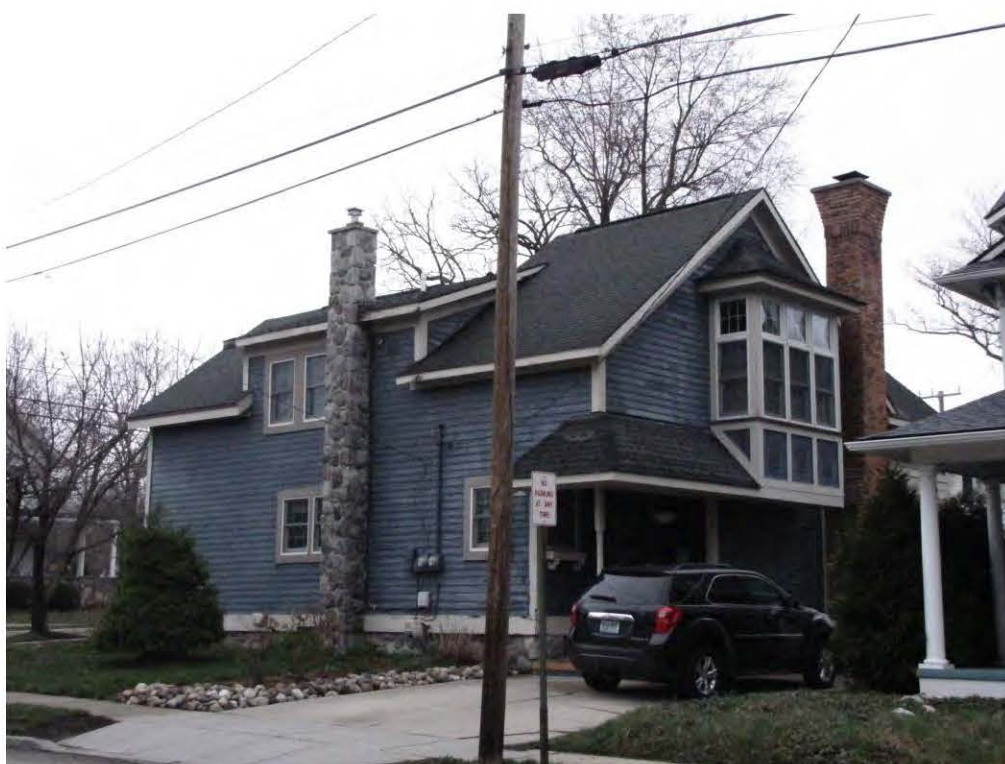
Rogers South 127_Looking Northwest
