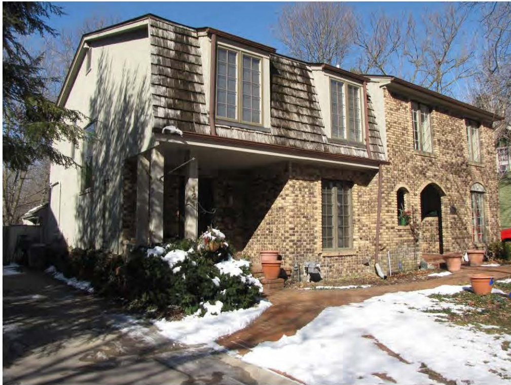
Rogers North 121-125_Looking Northwest
