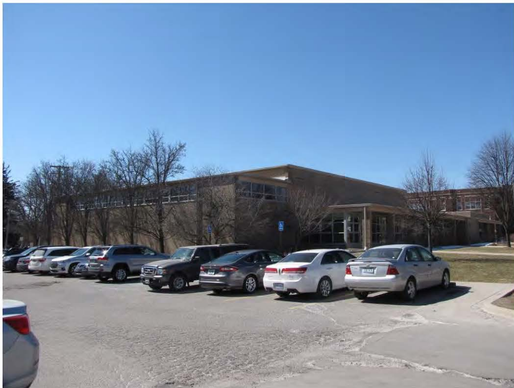
Main West 303_Looking Southwest
