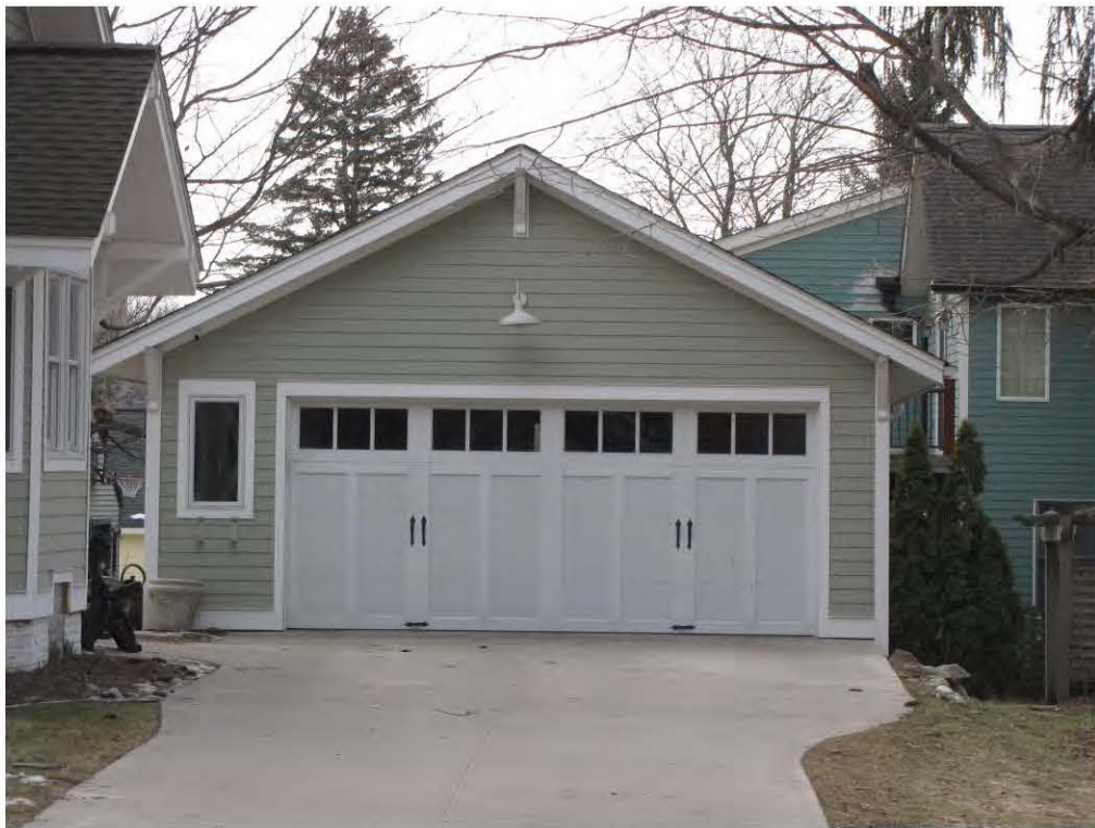
Cady West 487, Garage_Looking South
