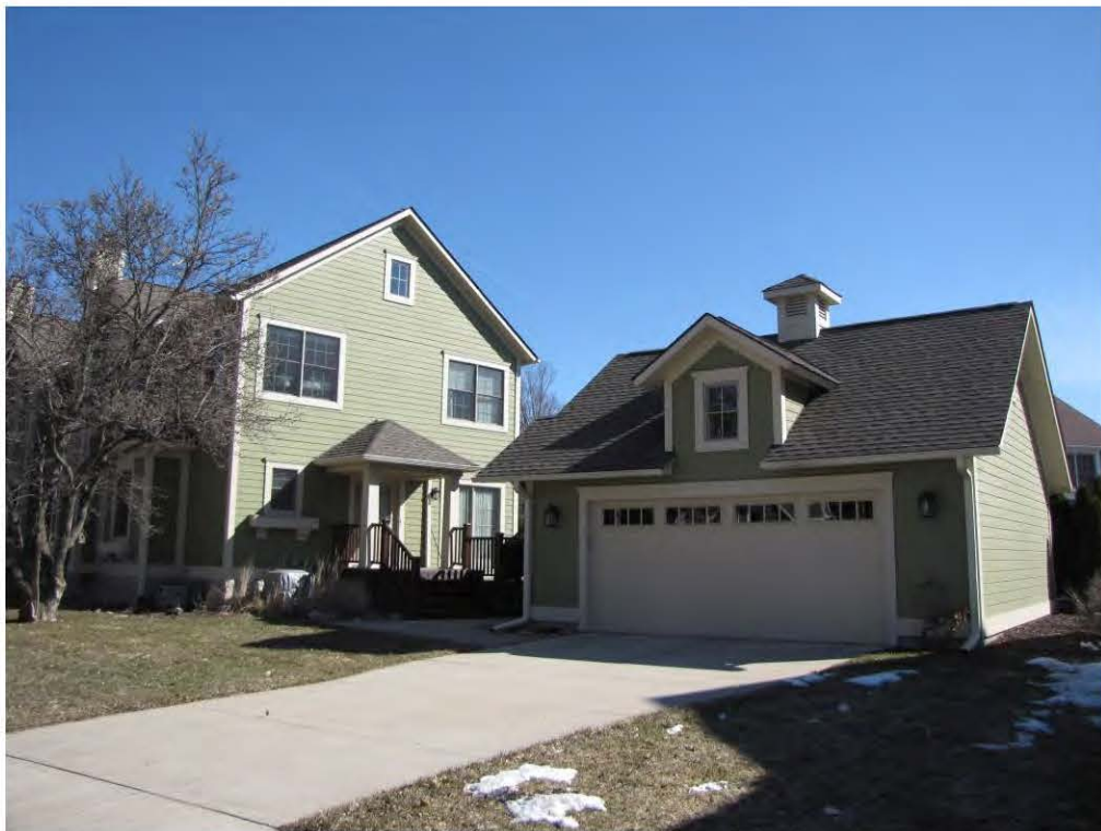
Randolph 413, Garage_Looking Northeast
