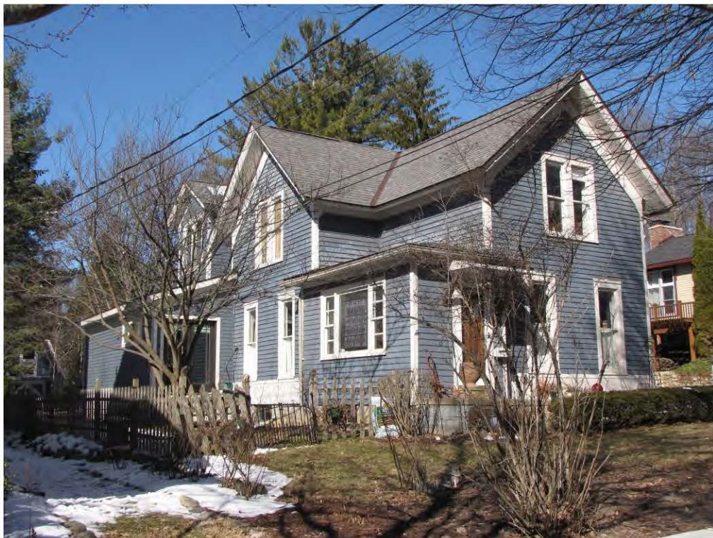
Rogers North 227_Looking Northwest
