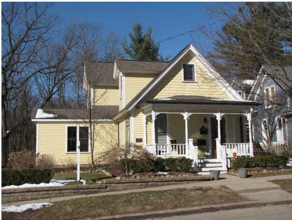
Rogers North 221_Looking Northwest
