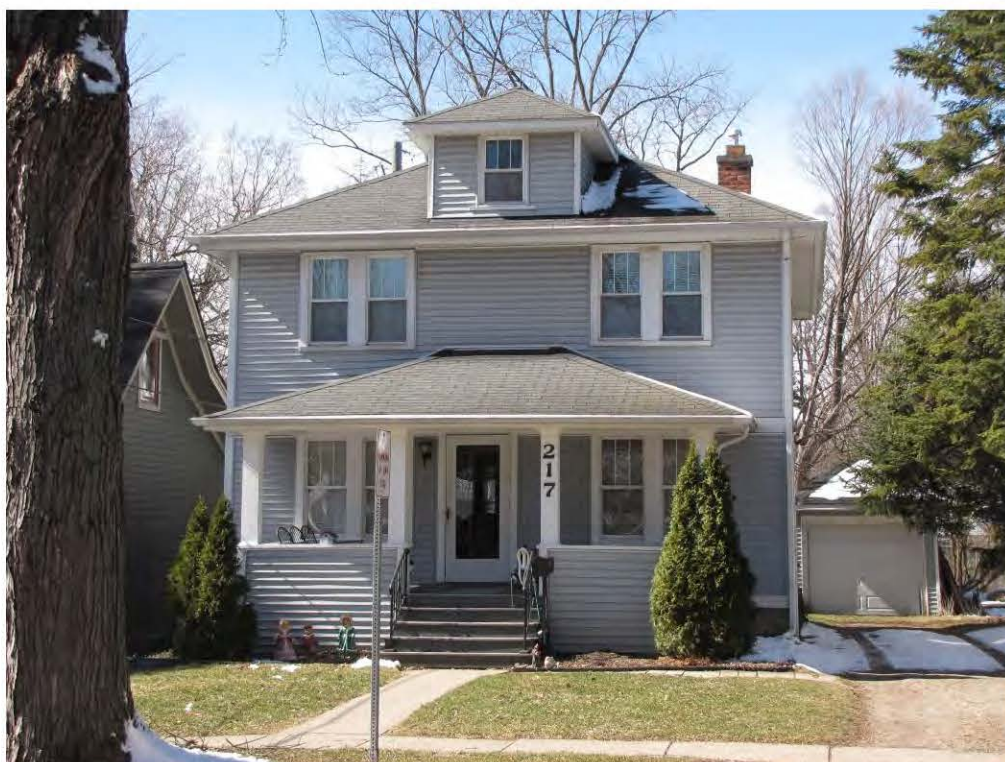
Linden 217, Garage_Looking West
