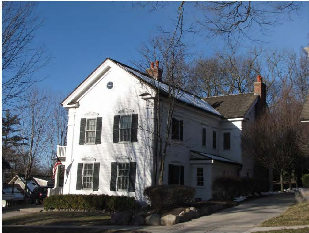
Rogers North 343_Looking Southwest
