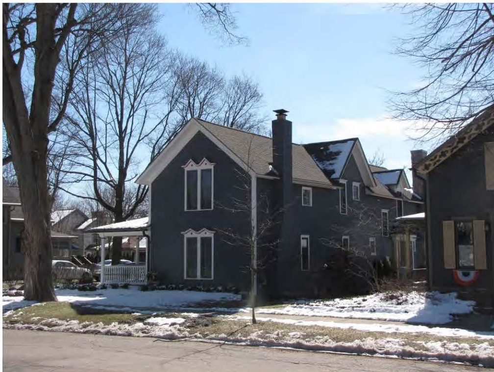
Dunlap West 523_Looking Southeast
