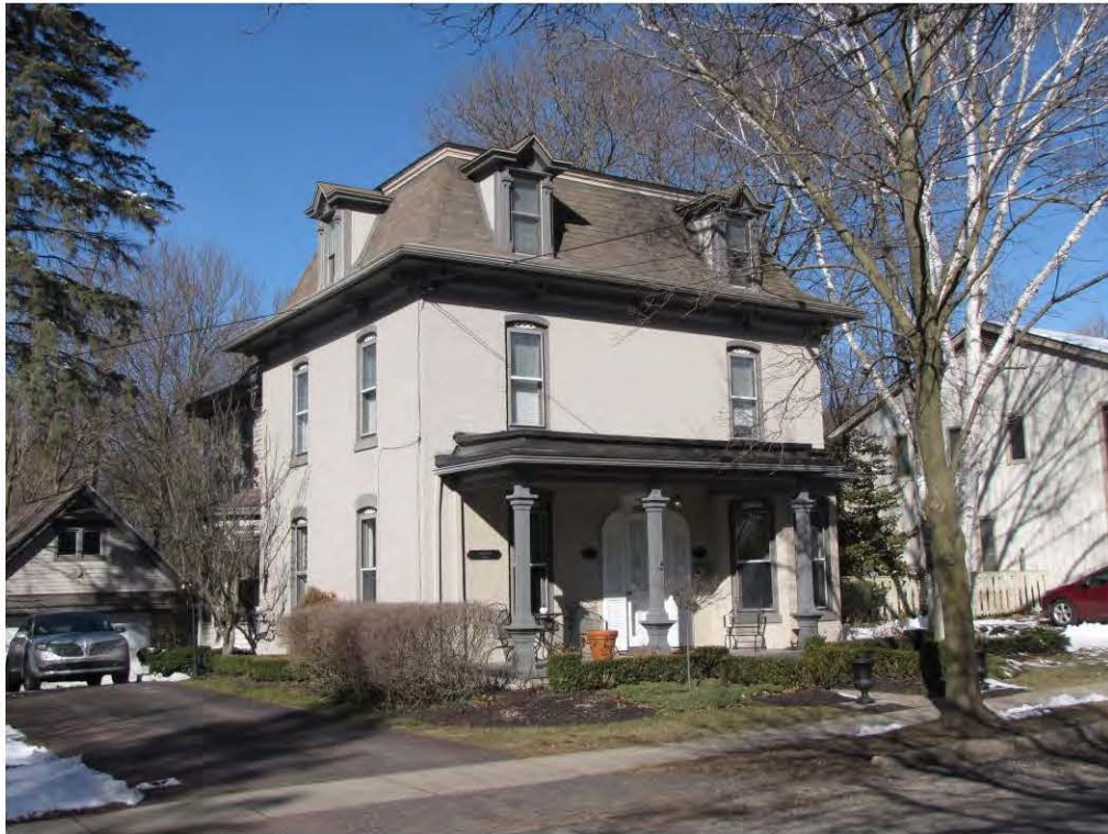
Rogers North 109_Looking Northwest
