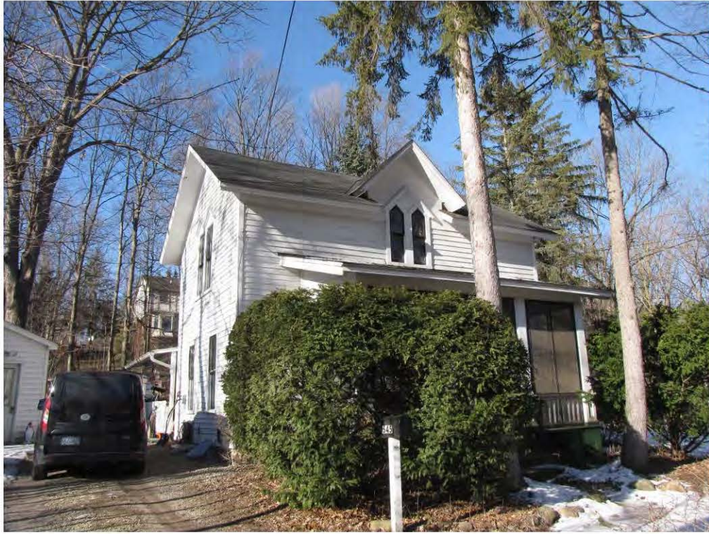
Randolph 545_Looking Southwest
