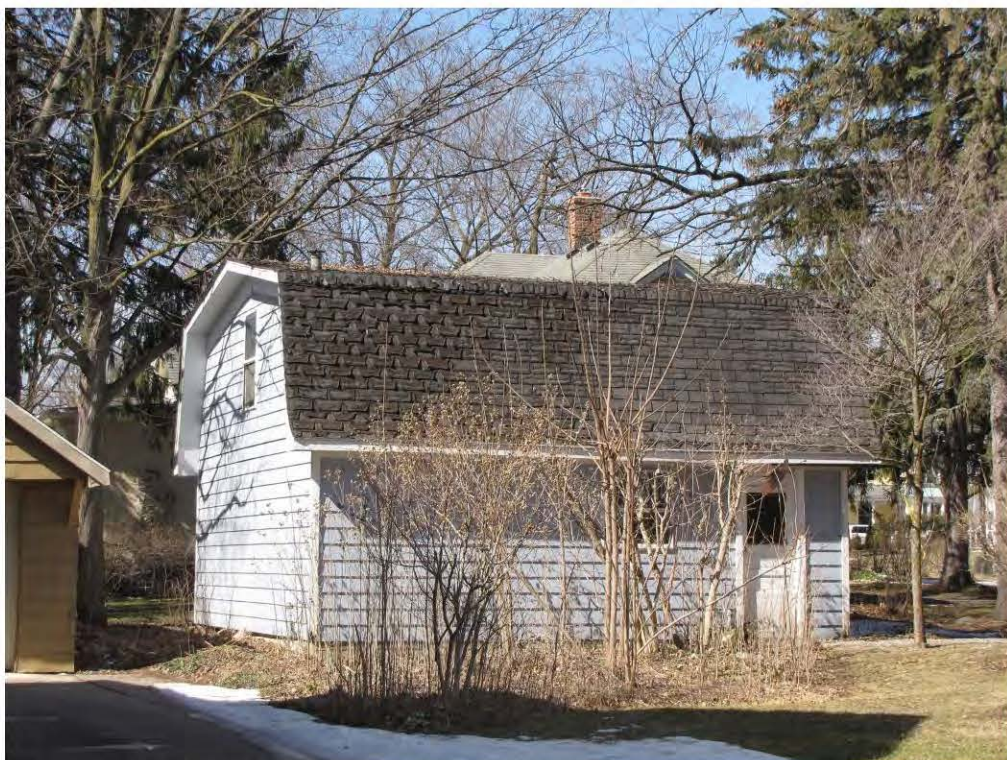
Dunlap West 305, Garage_Looking West
