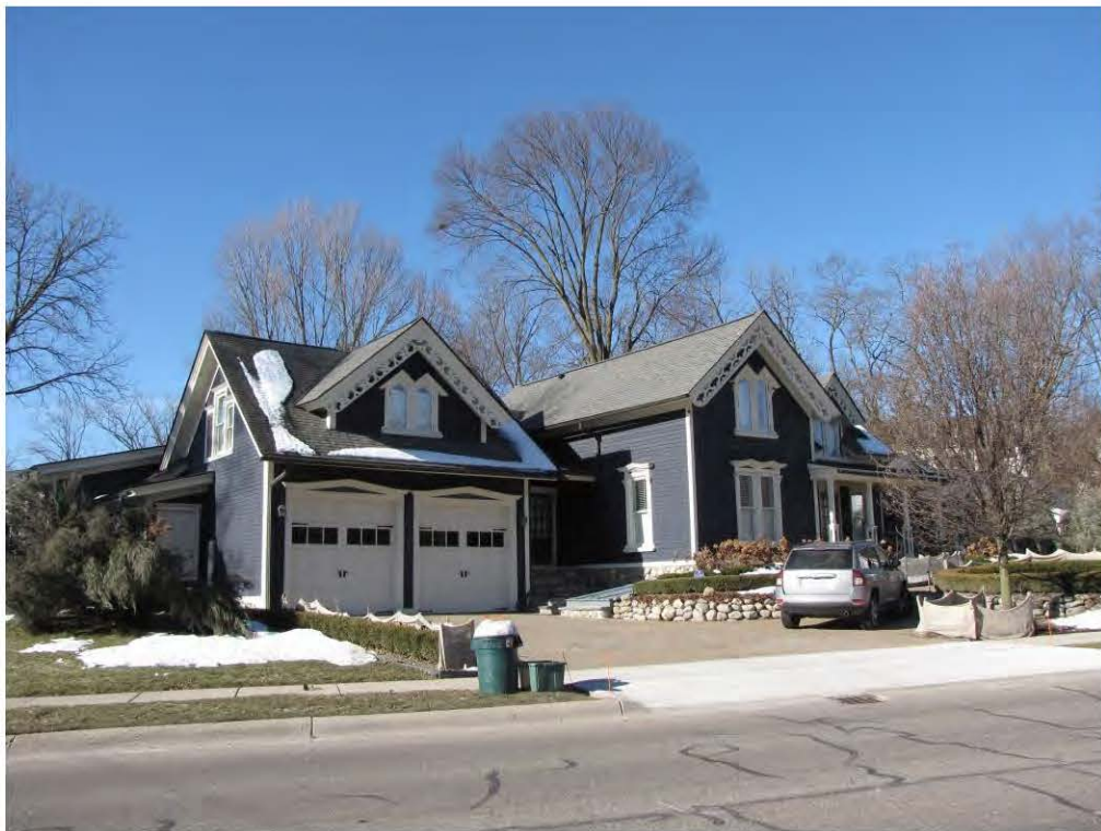
Randolph 521_Looking Southwest
