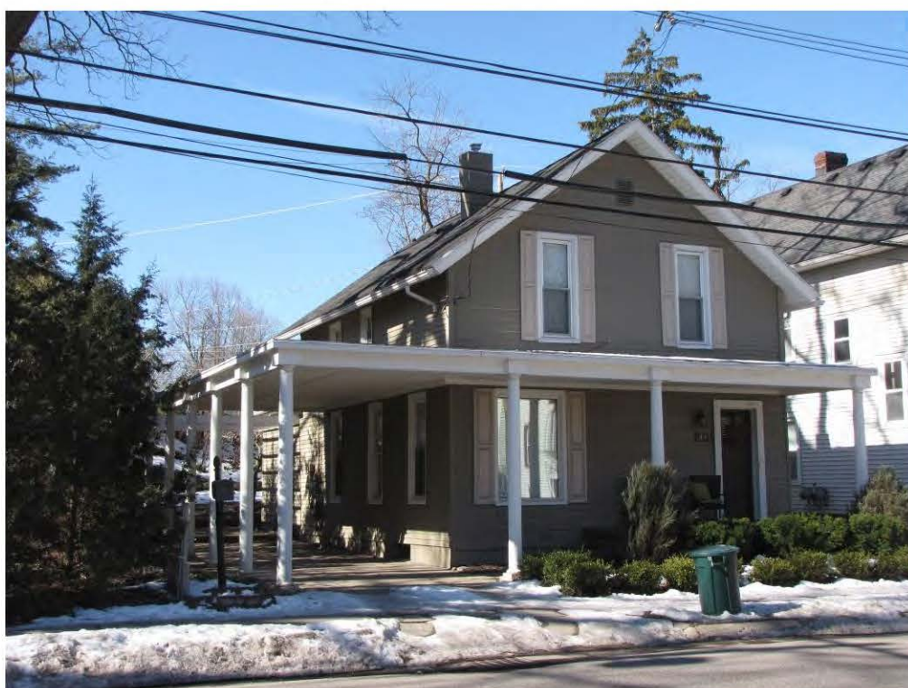
Randolph 317_Looking Southwest
