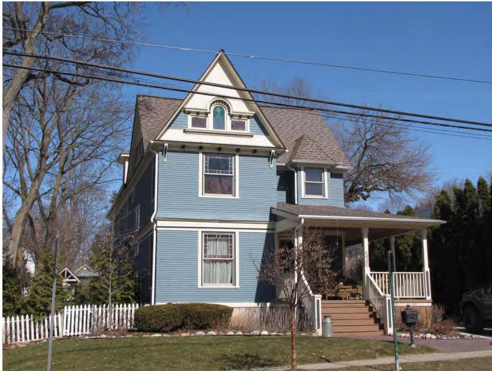
Main West 530_Looking North
