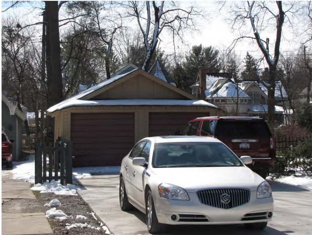
Main West 547, Garage_Looking South
