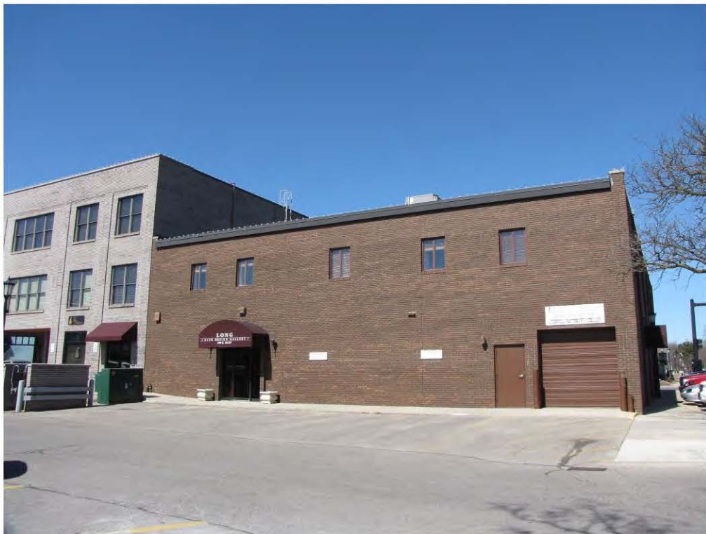
Main East 190_Looking Northwest
