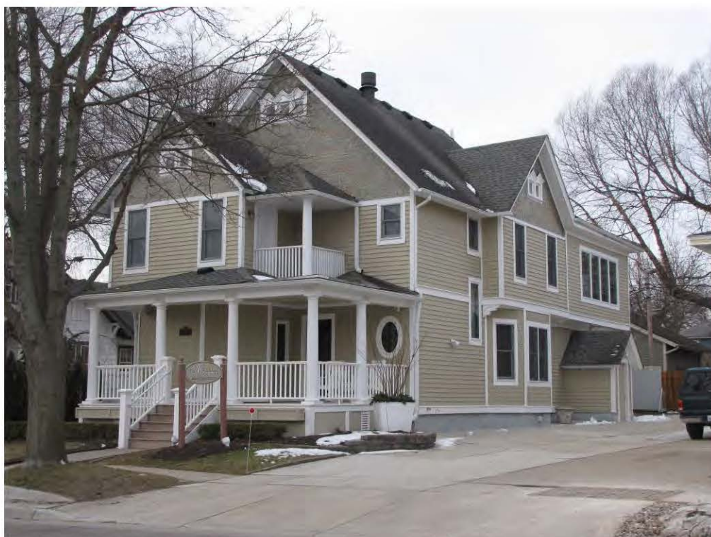
Wing North 117_ Looking Southwest
