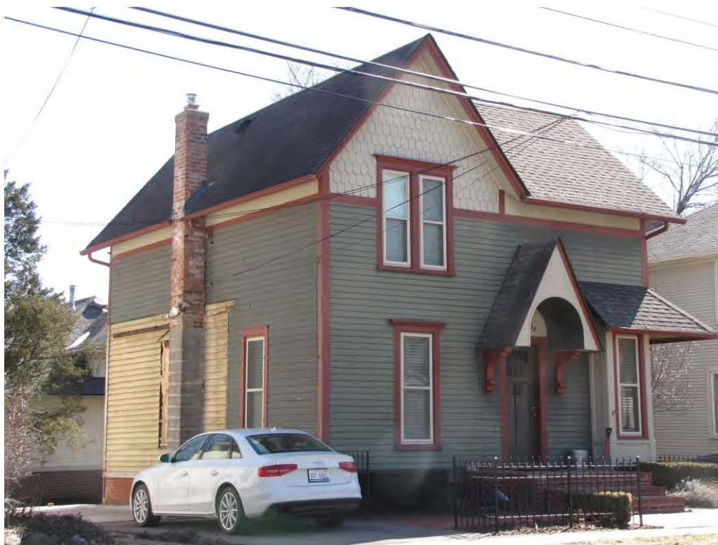
West 222_Looking Southeast
