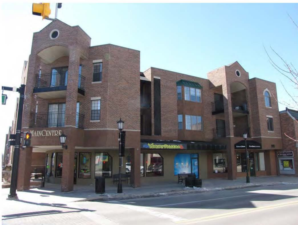
MainCentre 150_Looking Southwest
