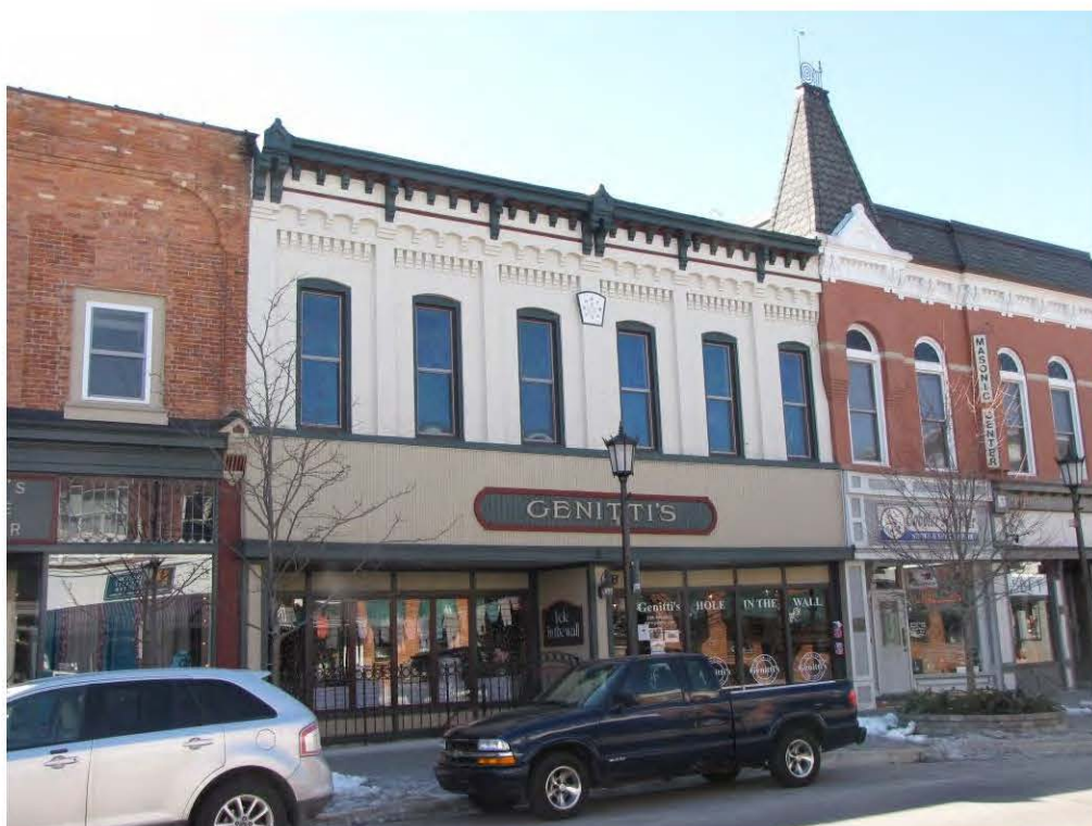
Main East 108-110_Looking Southeast
