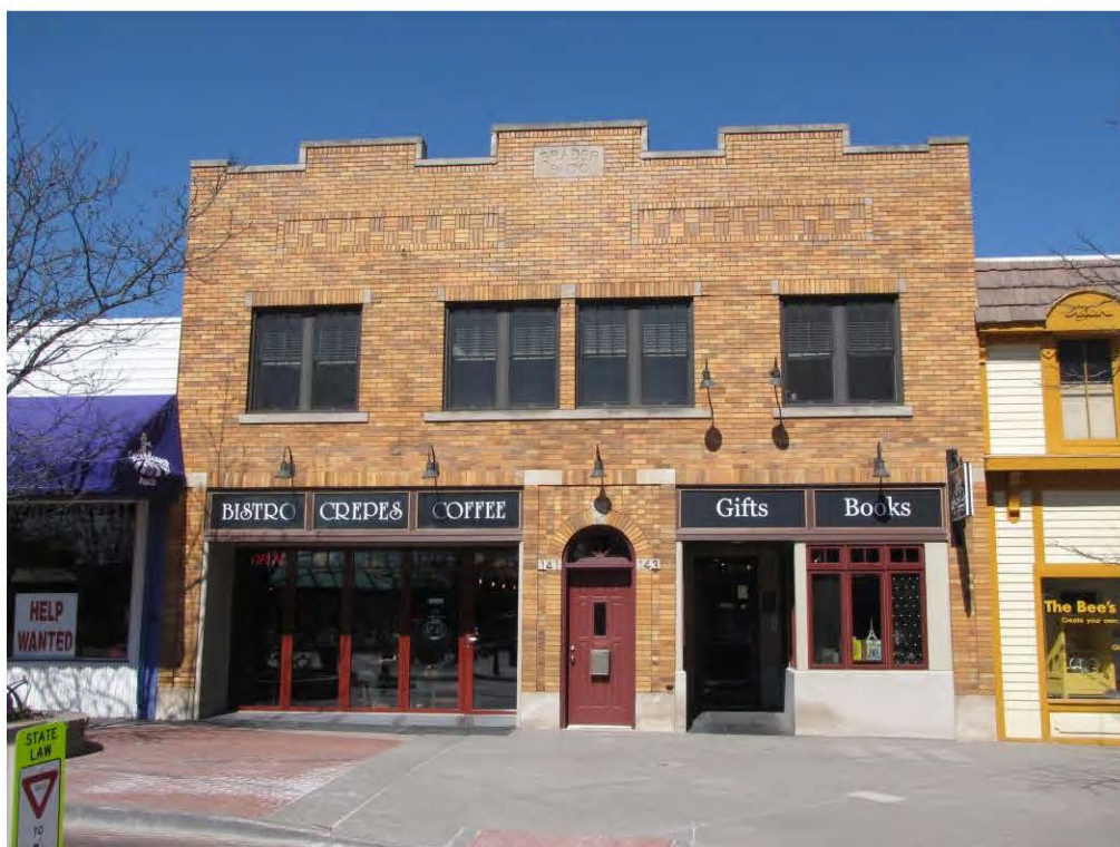
Main East 141-143_Looking North
