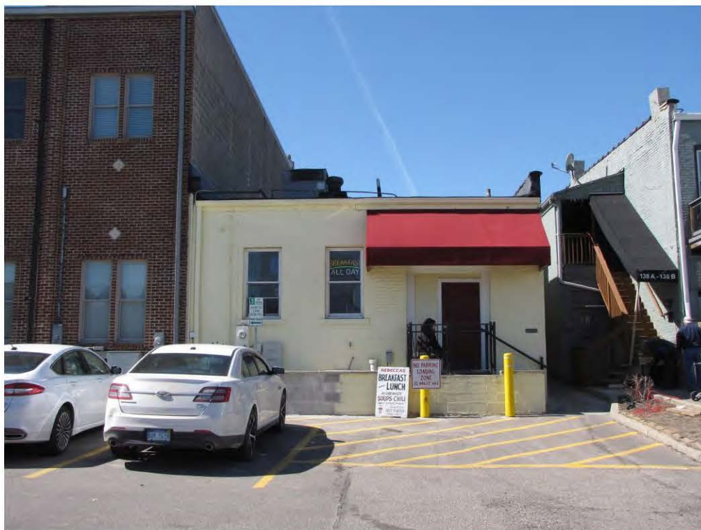
Center North 134_Looking West
