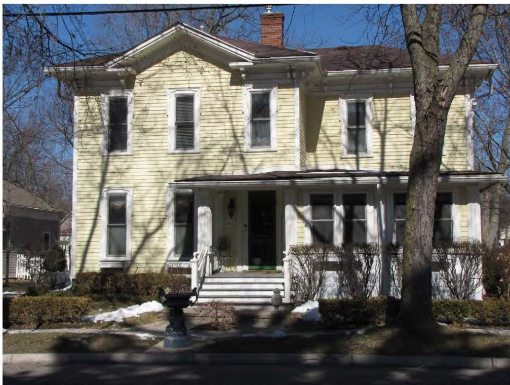
Main West 502_Looking North
