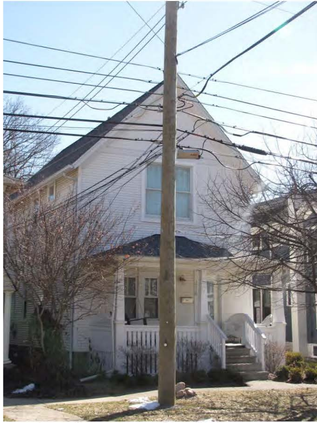
West 216_Looking Southeast
