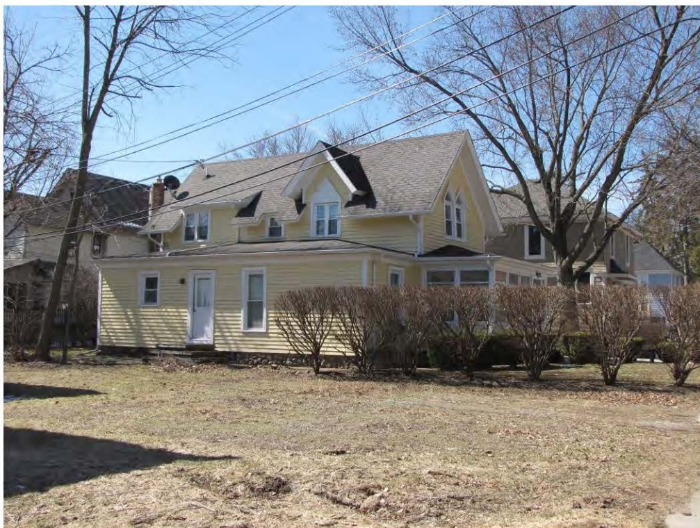
Dunlap West 211_Looking Southwest
