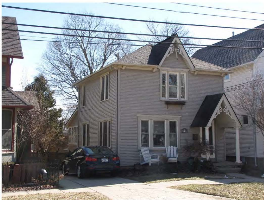
West 218_Looking Southeast
