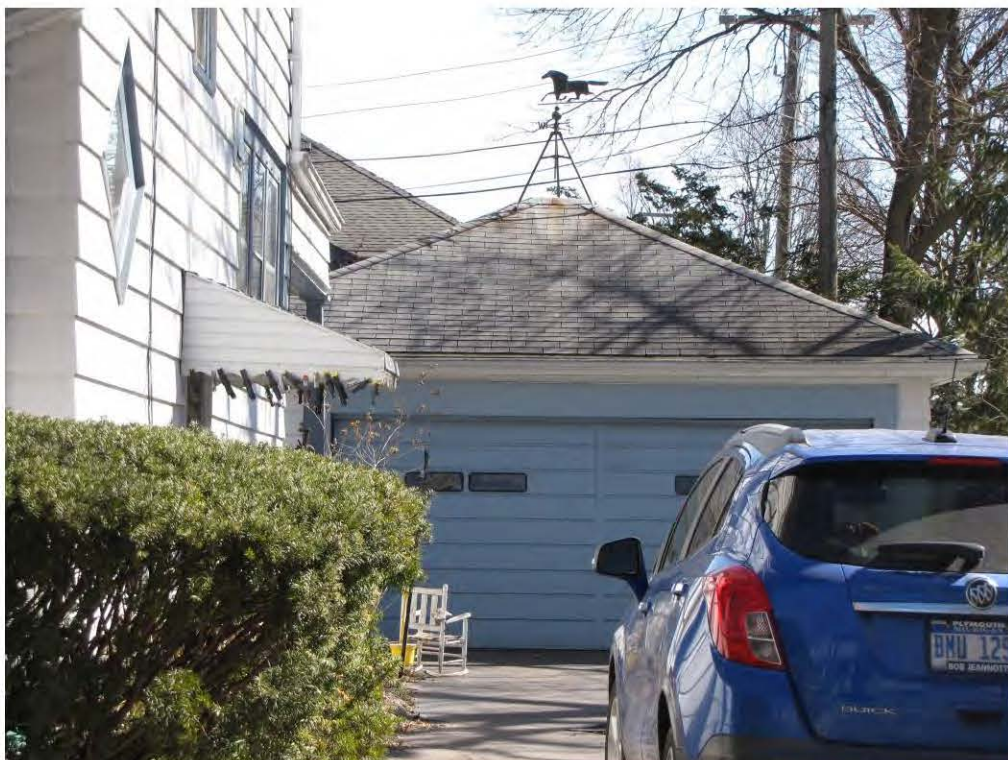
West 114, Garage_Looking East
