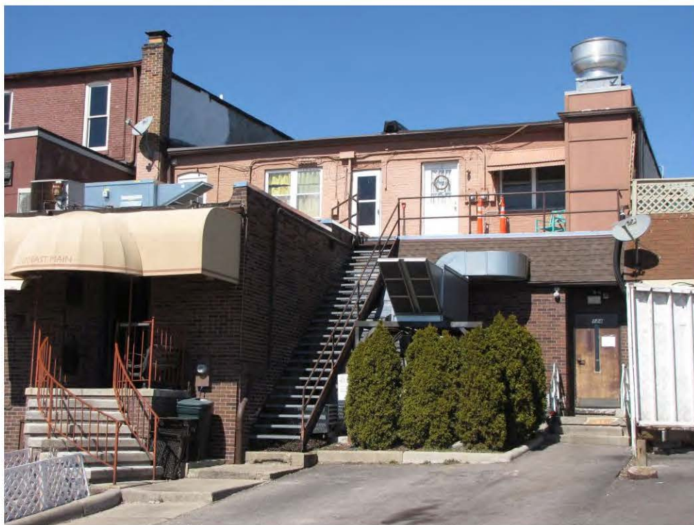
Main East 120-124_Looking Northwest
