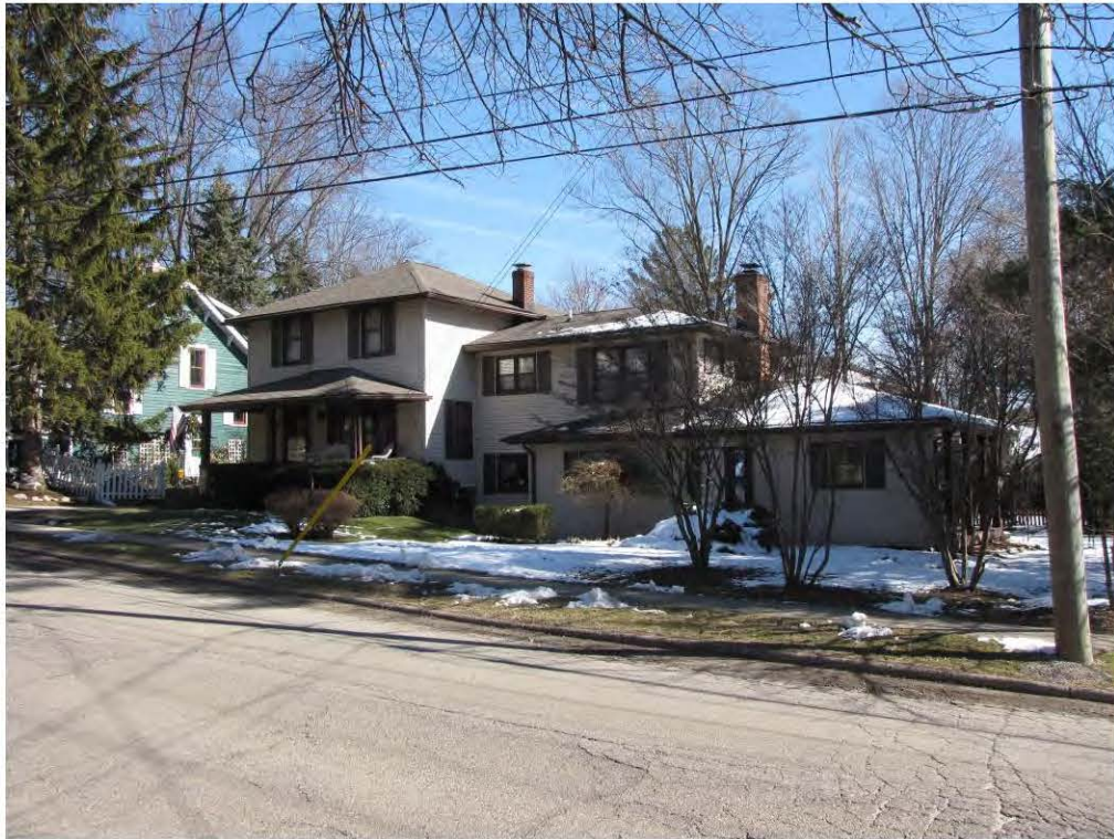
Rogers North 230_Looking Northeast
