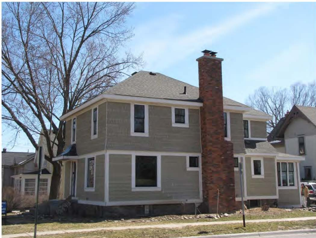
Dunlap West 217_Looking Southeast
