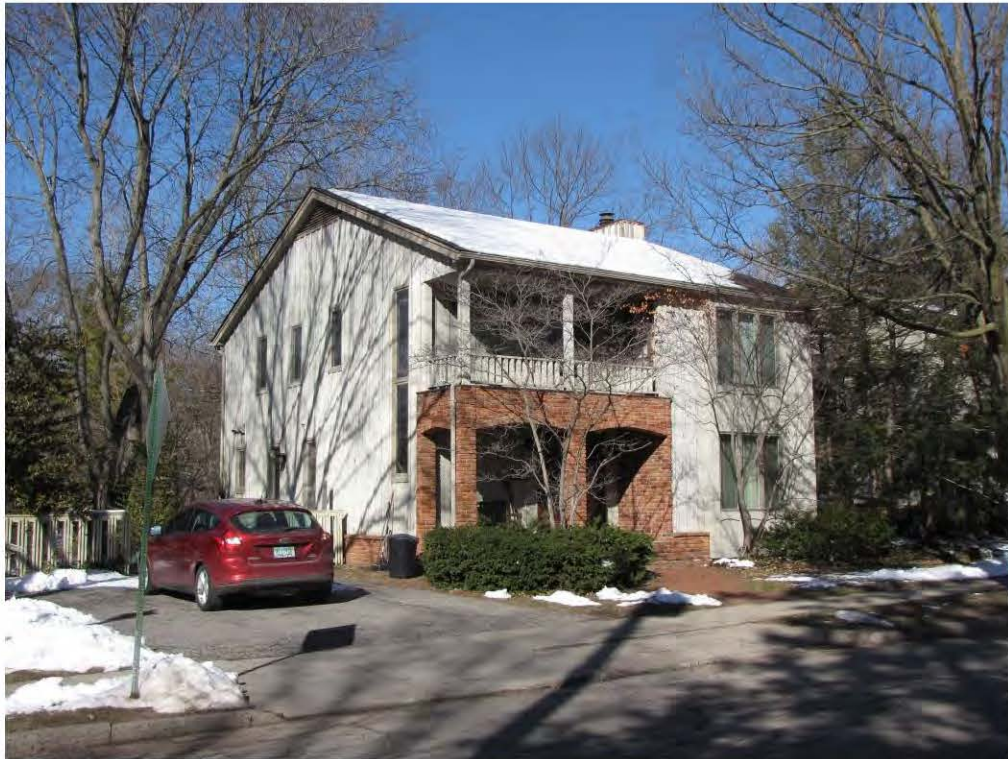
Rogers North 117_Looking Northwest
