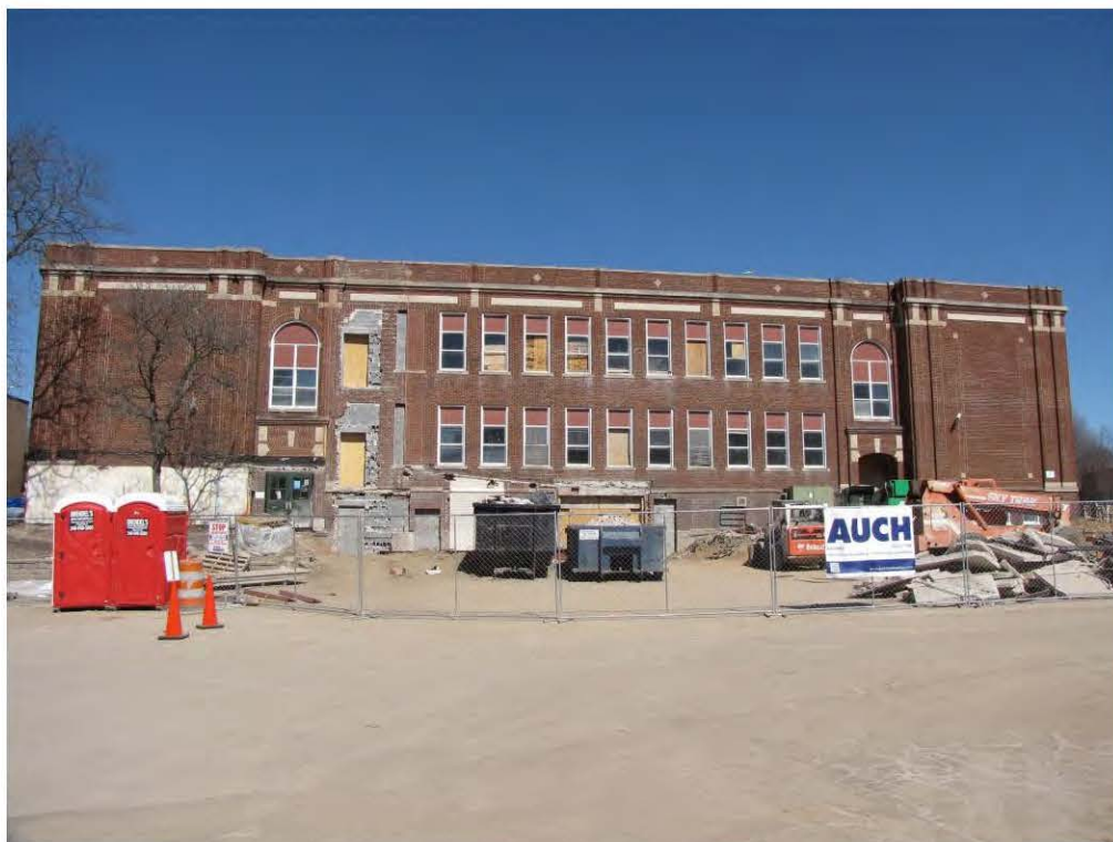
Main West 411_Looking North
