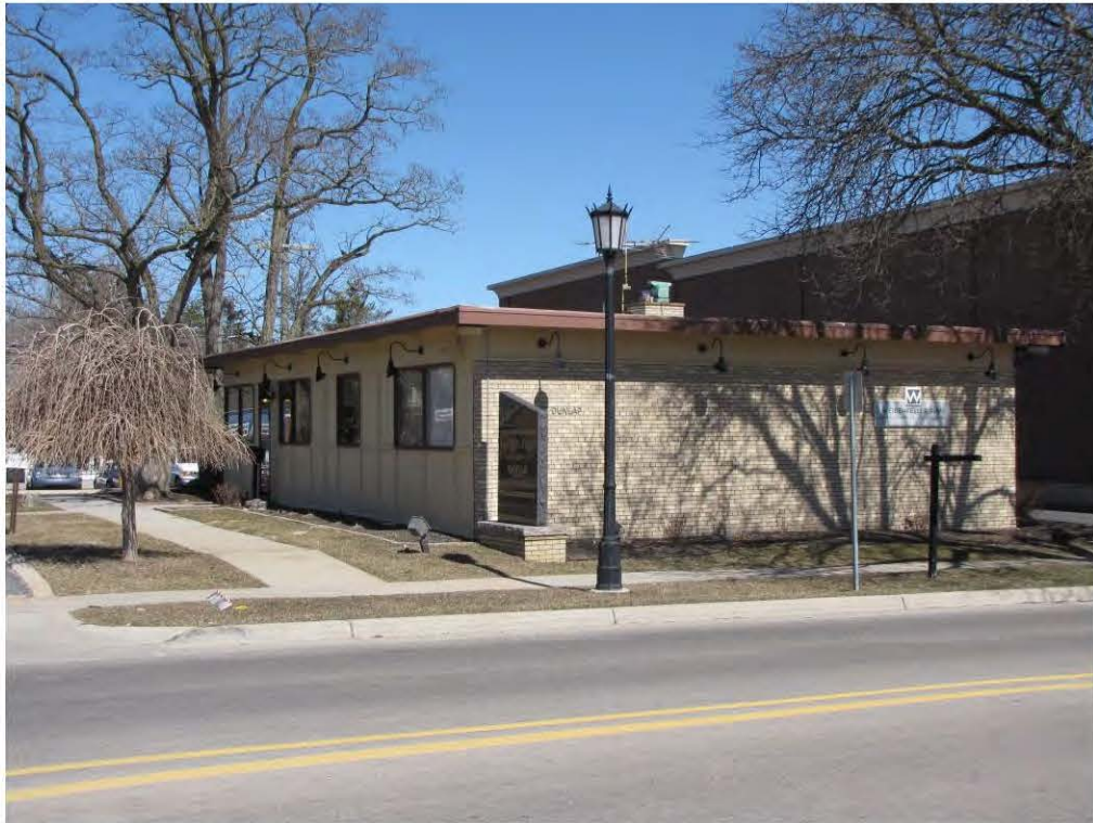
Dunlap East 115_Looking Northeast
