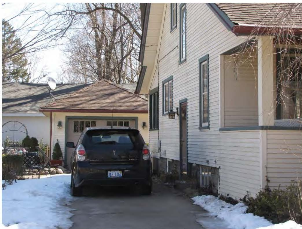
Linden 118, Garage_Looking East
