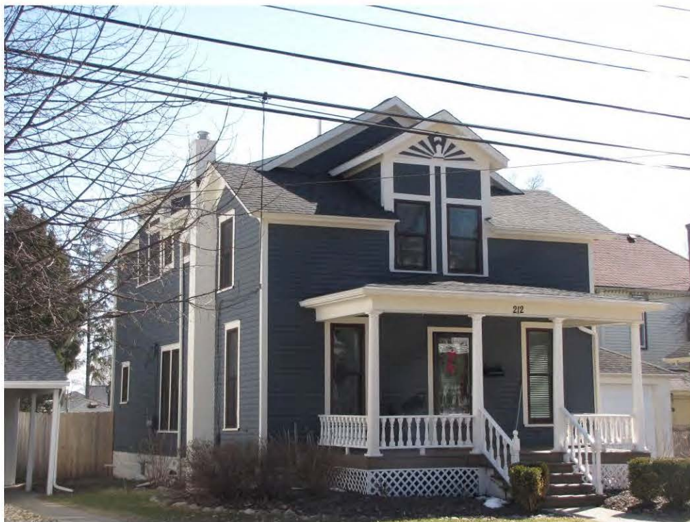
West 212_Looking Southeast
