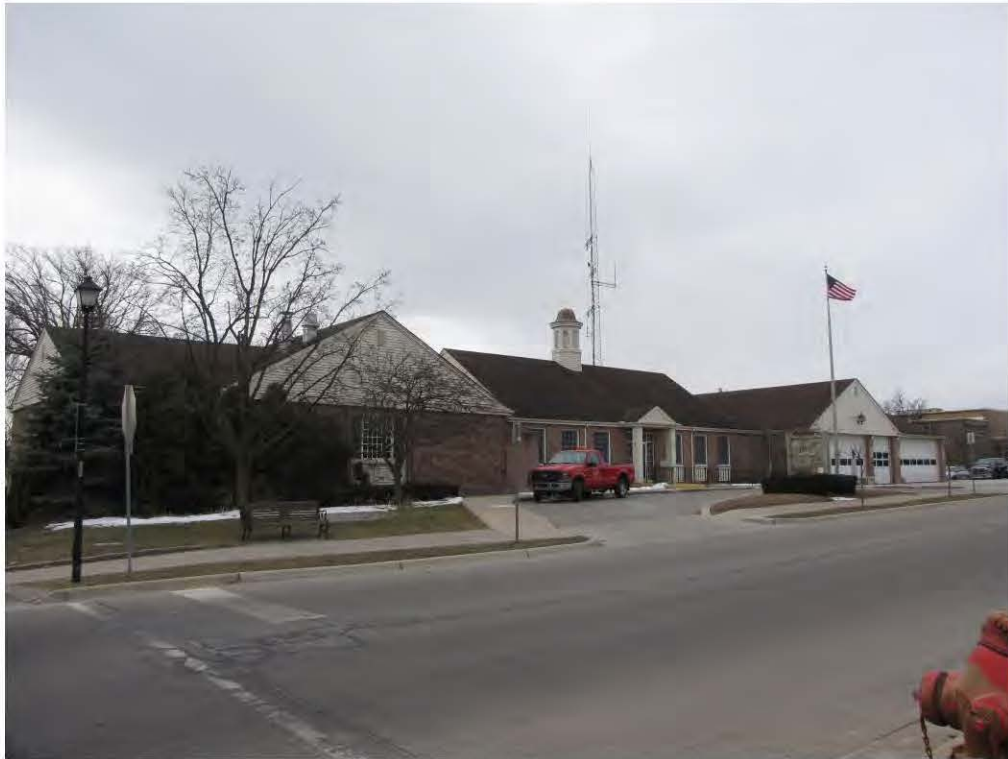
Main West 215_Looking Southwest
