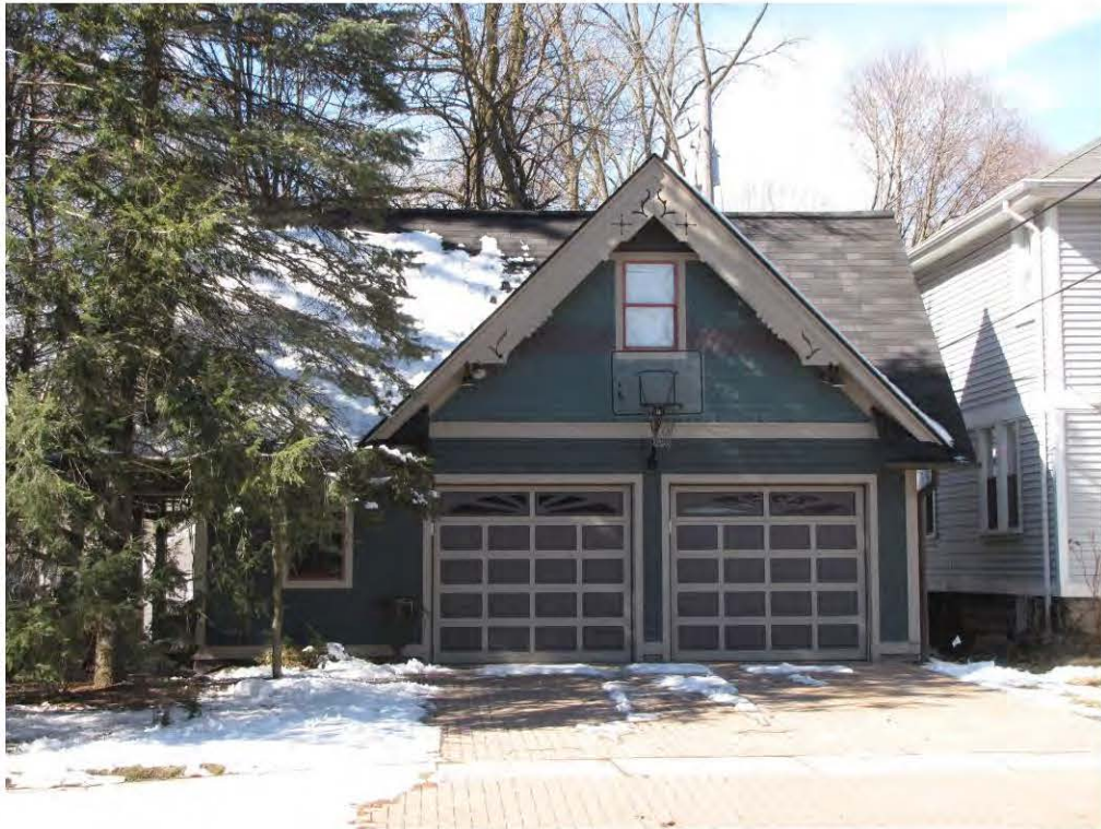
Dunlap West 504, Garage_Looking West
