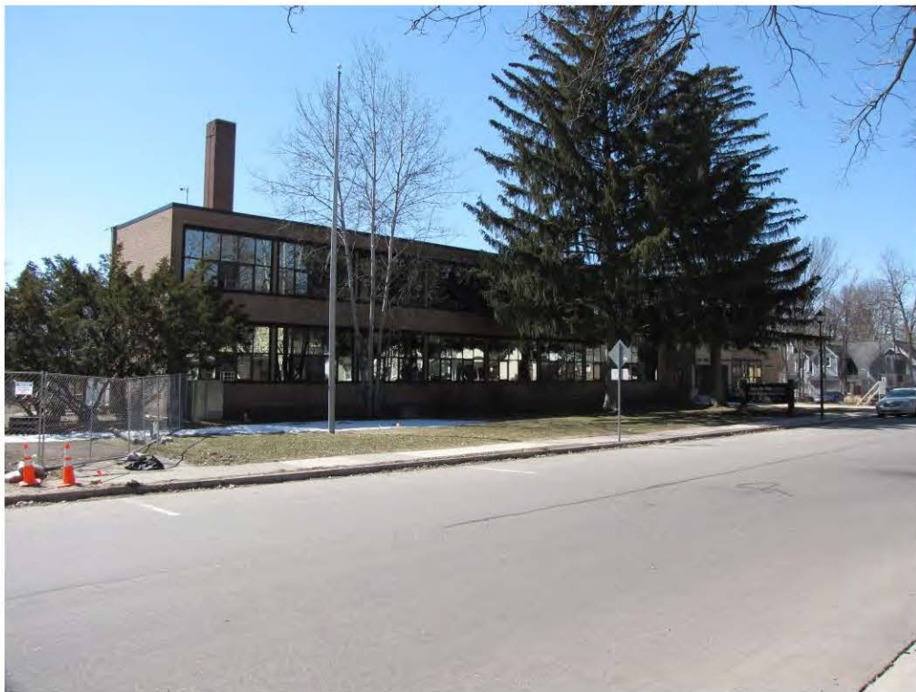
Main West 501_Looking Southwest
