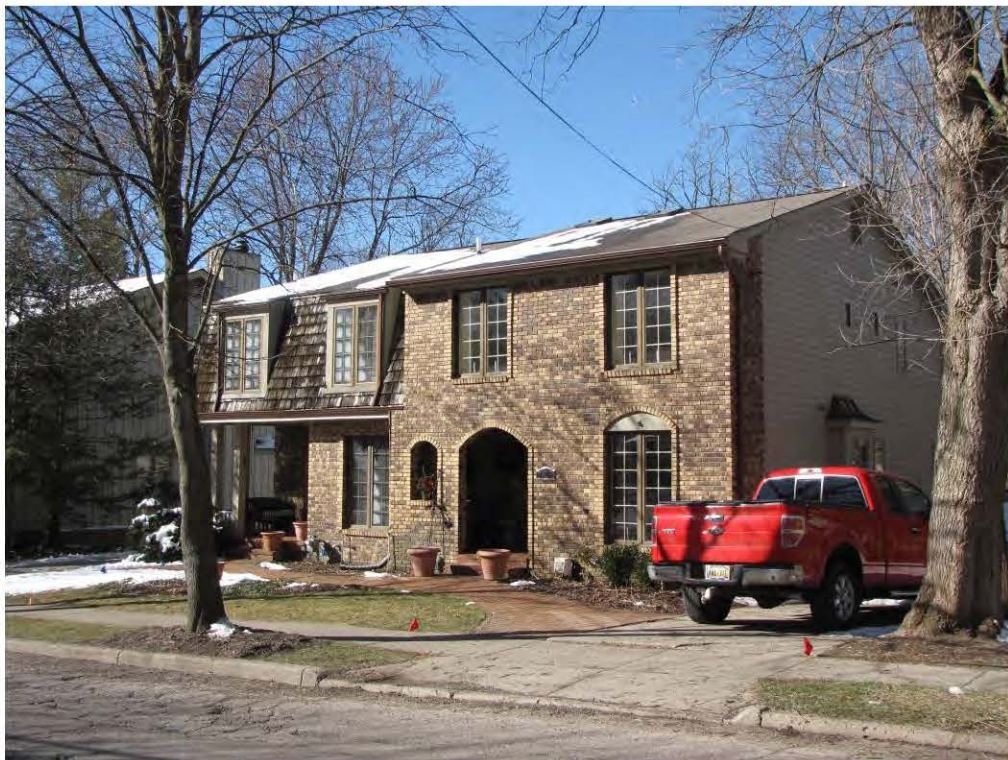
Rogers North 121-125_Looking Southwest
