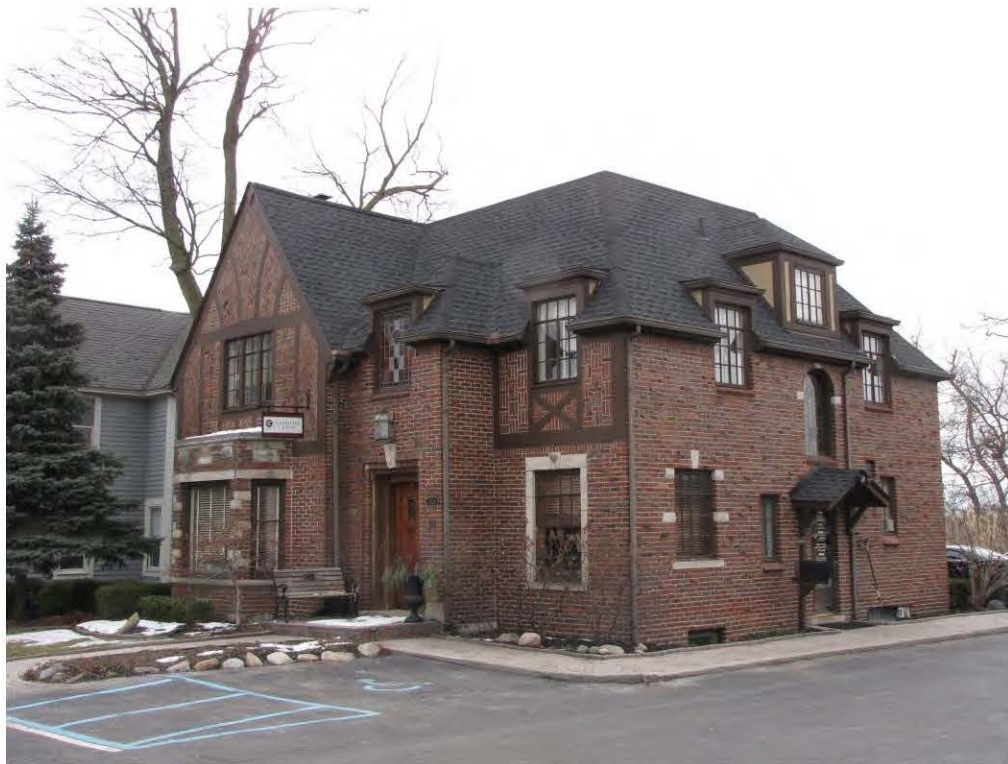
Main East 324_Looking Southeast
