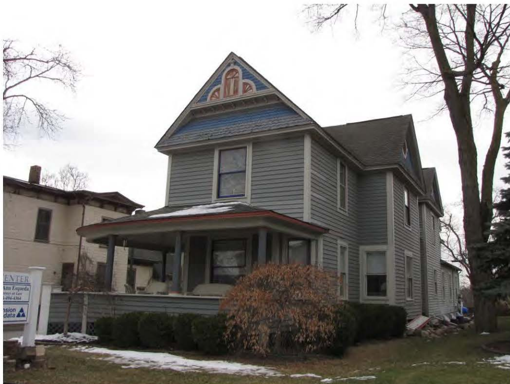
Main East 332_Looking Southeast
