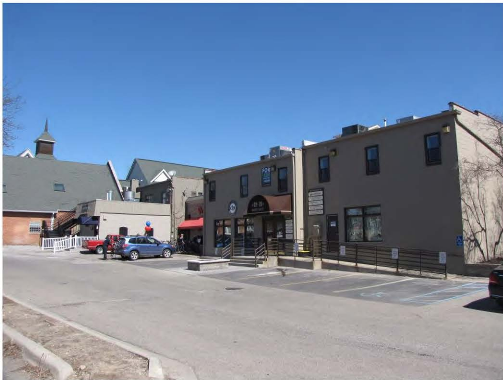
Center North 109-115_Looking Northeast
