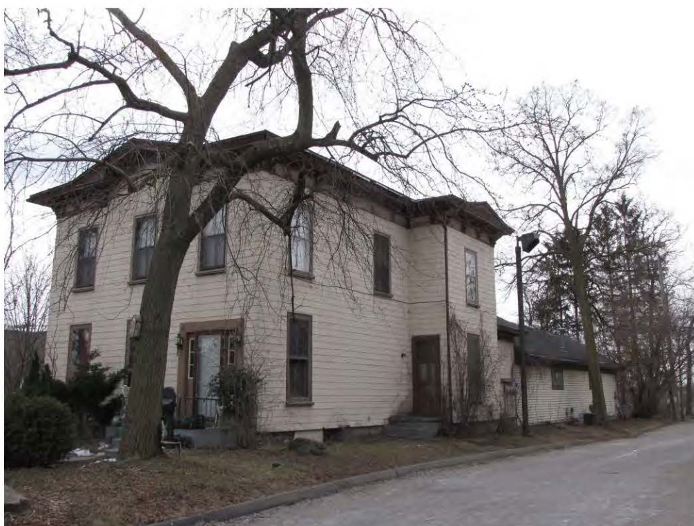
Main East 342_Looking Southeast
