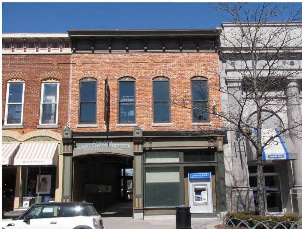
Main East 125_Looking North
