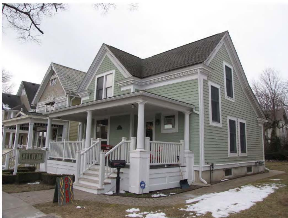
Wing North 125_ Looking Southwest
