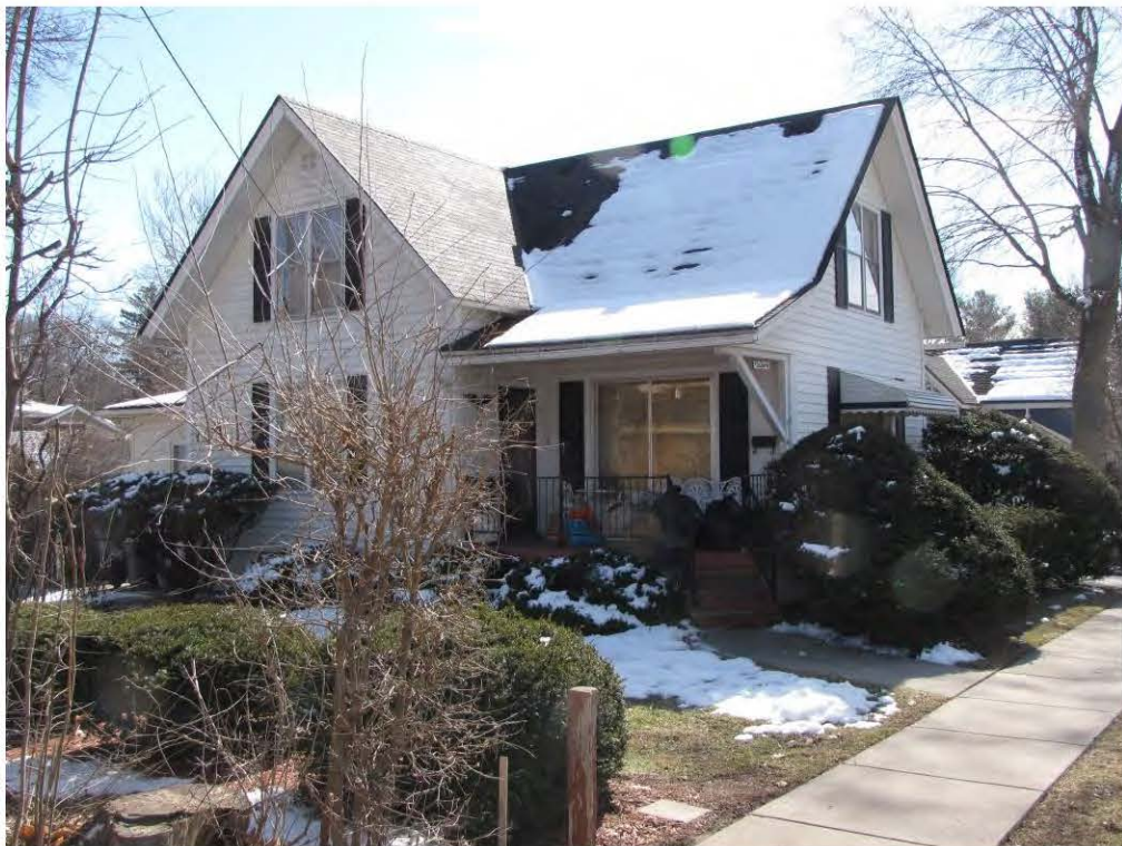
Rogers South 117_Looking Southeast
