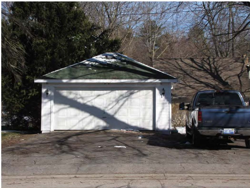
Rogers North 101, Garage_Looking North
