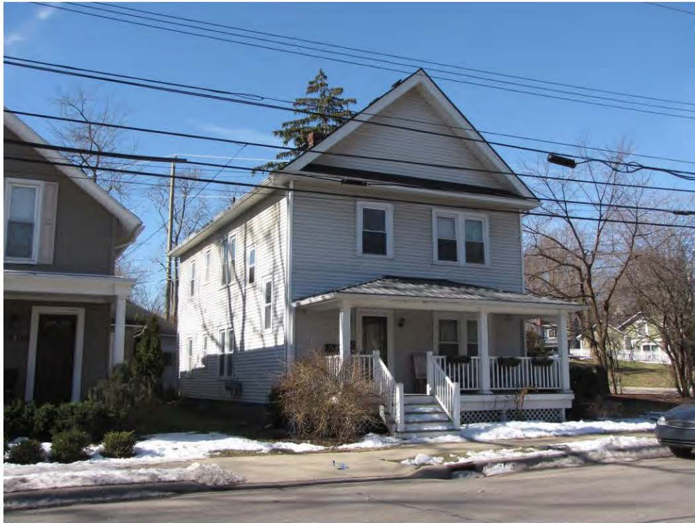
Randolph 319-321_Looking Southwest
