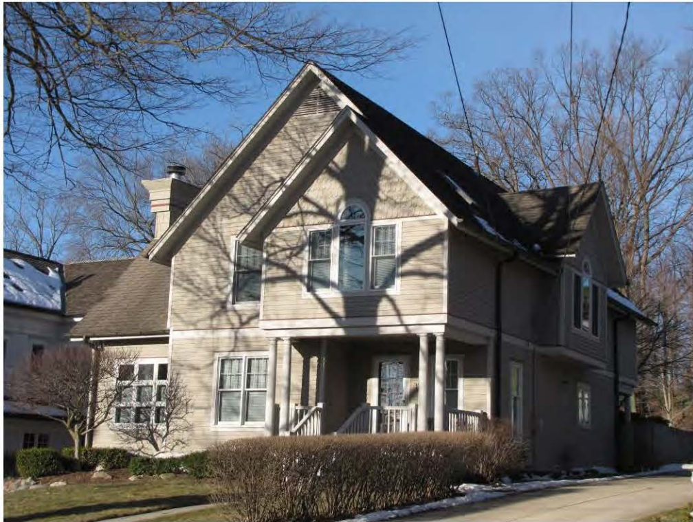
Rogers North 353_Looking Southwest
