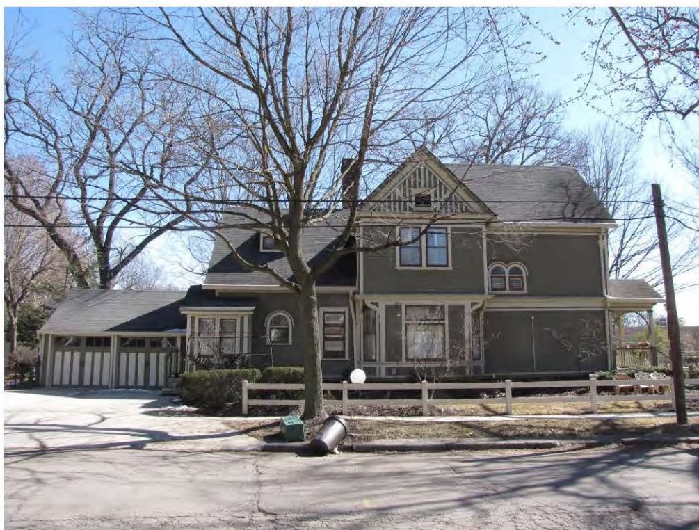
Main West 418_Looking East
