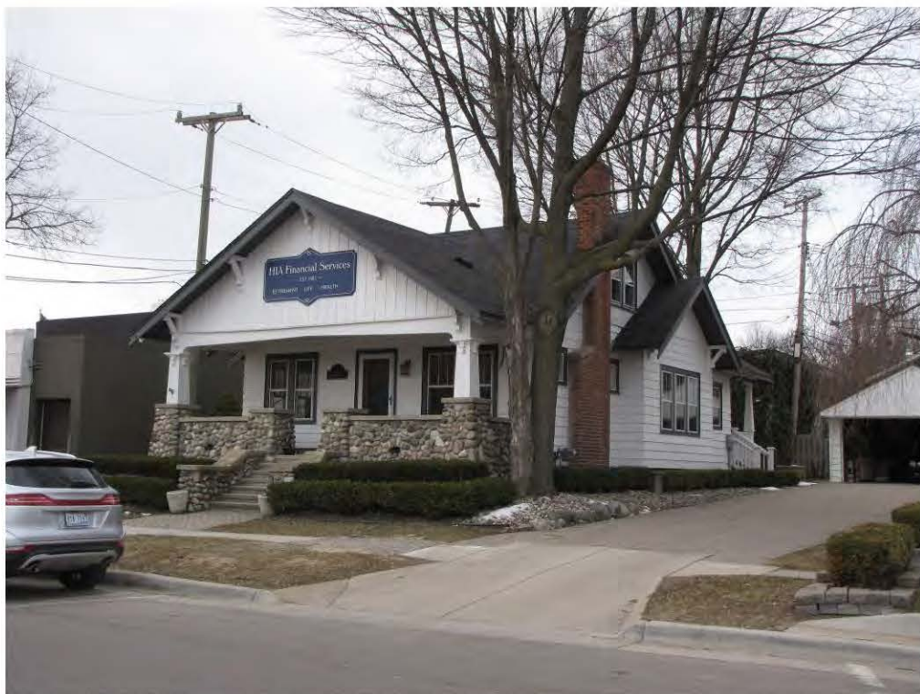
Wing North 111_Looking Southwest
