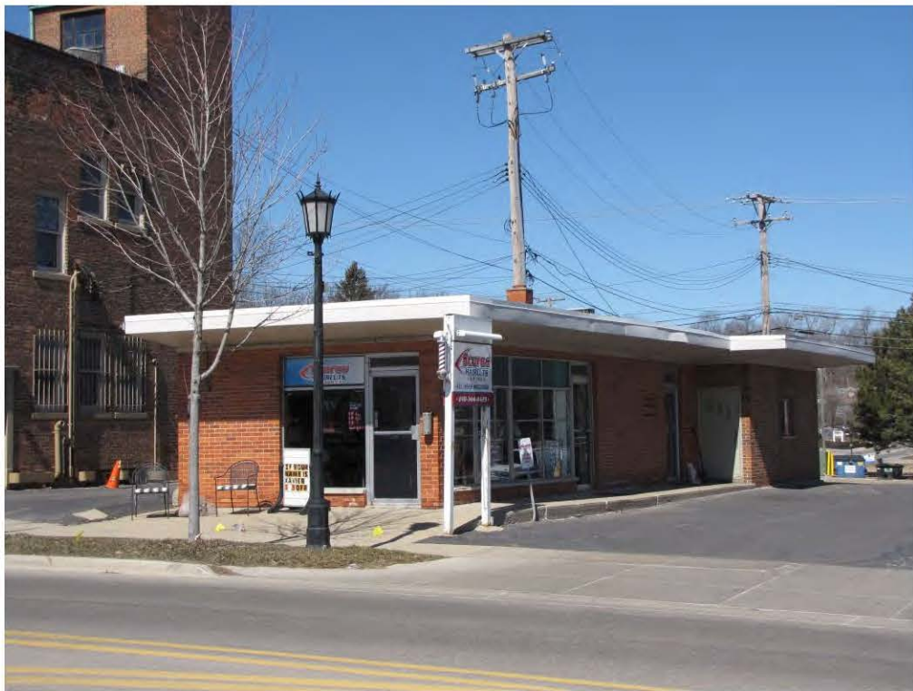
Dunlap East 111_Looking Northwest
