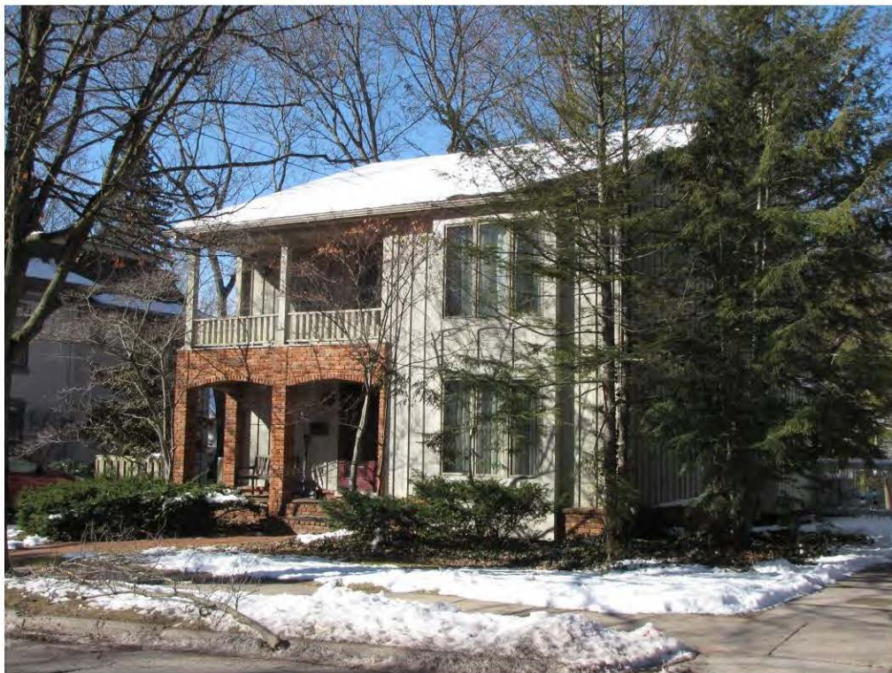
Rogers North 117_Looking Southwest
