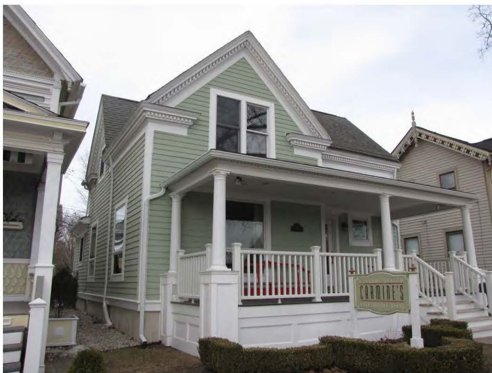
Wing North 125_ Looking Northwest
