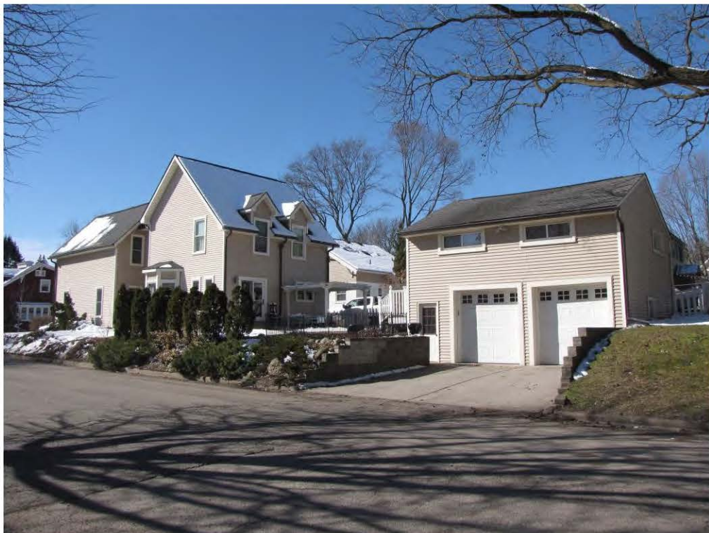
Dubuar 404, Garage_Looking Southwest
