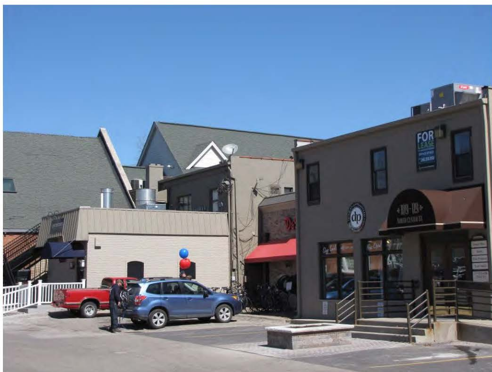
Center North 135-137_Looking Northeast
